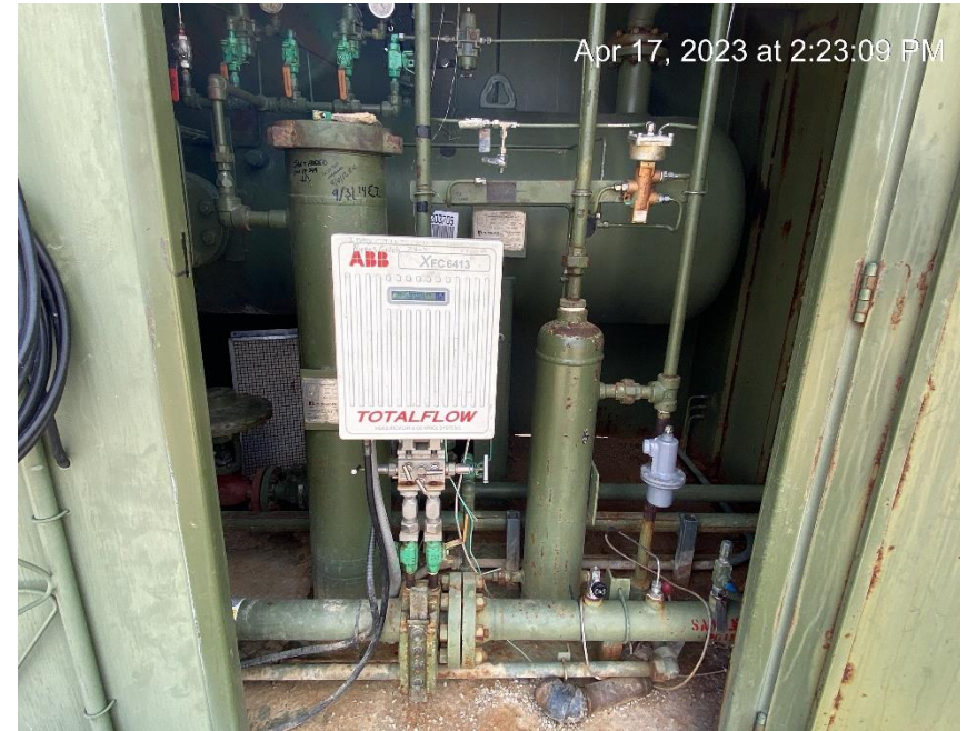
Gas meter calibration card not visibly displayed
