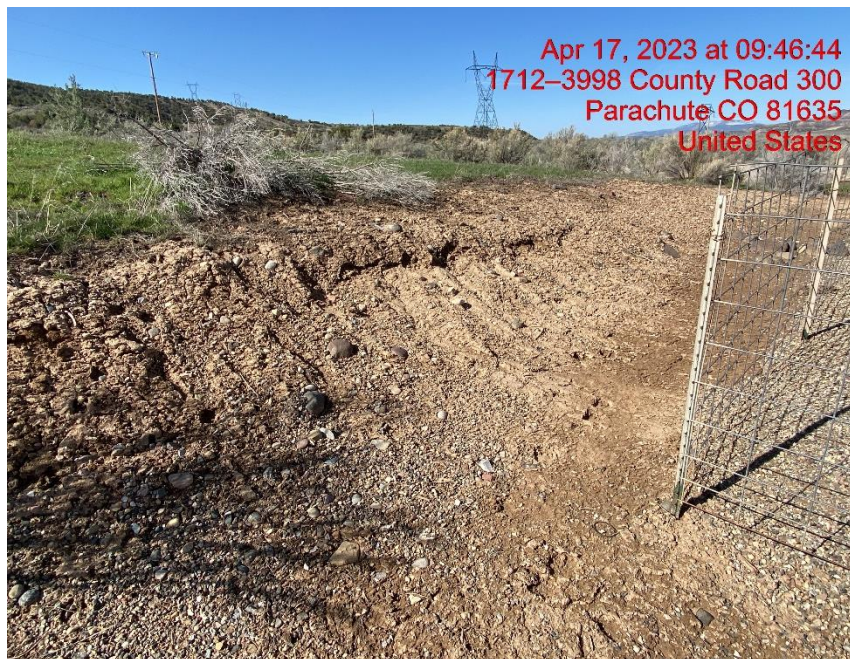
Rill Erosion onto Location – Photo #02233
