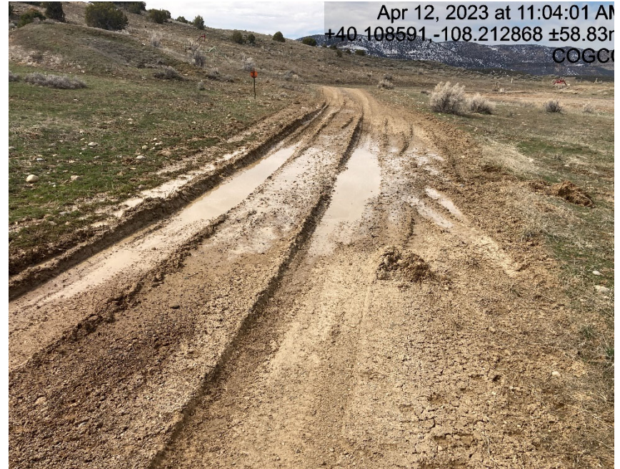
Access road lacks sufficient BMP's
