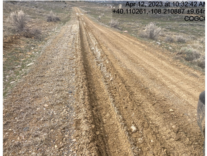
Access road lacks sufficient BMP's
