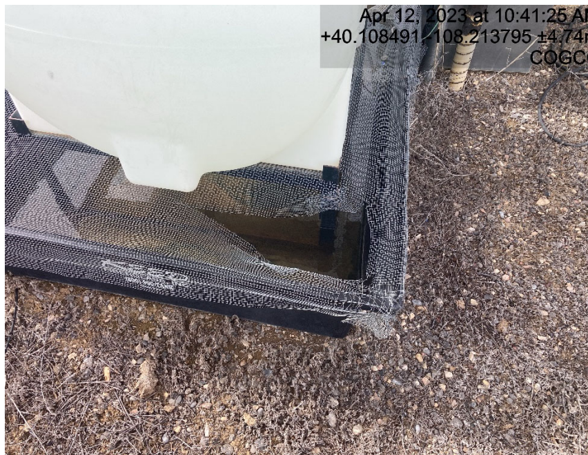
Chemical tank containment is full and wildlife protection insufficient
