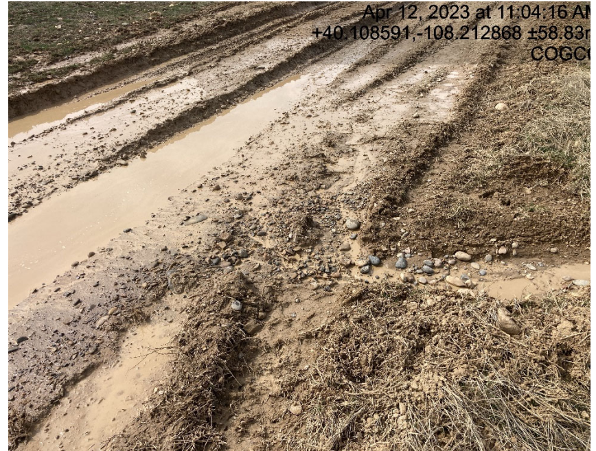
Access road lacks sufficient BMP's
