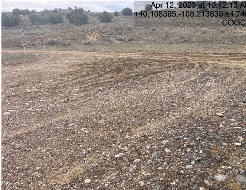
Lack of stabilization/compaction
