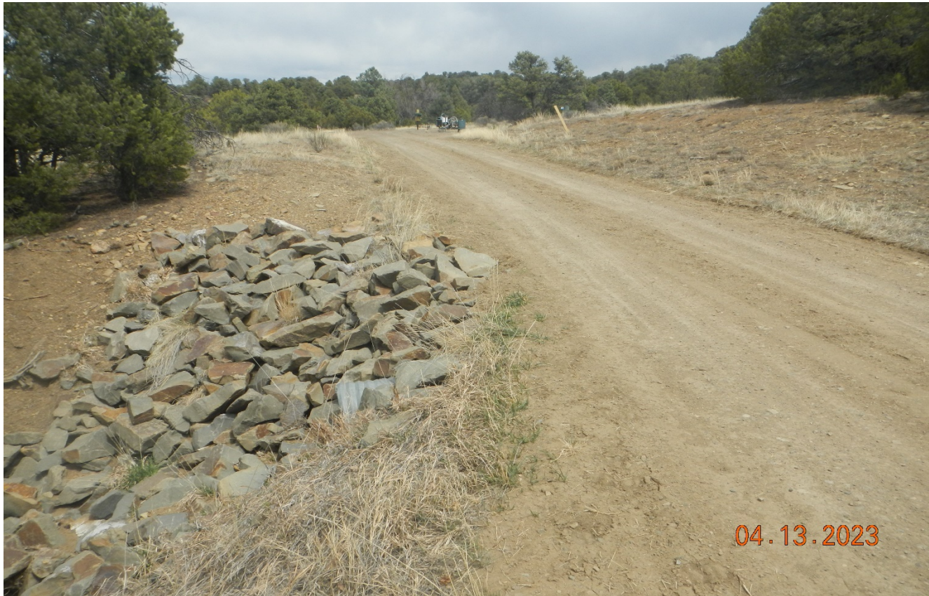
Photo 1. Facing northeast along the access road toward the wellsite.
