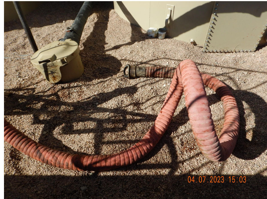
Photo 8. Photo taken from within the secondary containment, illustrating a hose being stored within secondary containment. COGCC staff communicated that this is considered unused equipment and needs to be removed.
