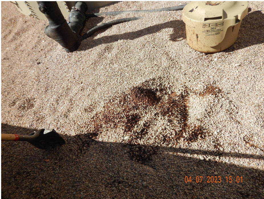
Photo 7. Photo taken from within the secondary containment, illustrating oily waste. Remove and properly dispose fluids from within the secondary containment.
