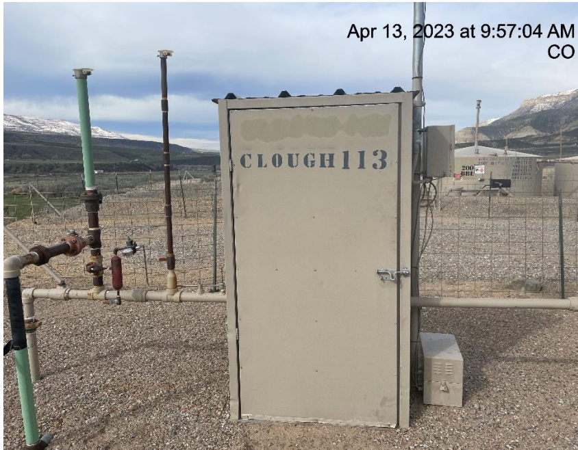
Photo # 5346 Meter calibration info not conspicuously posted
