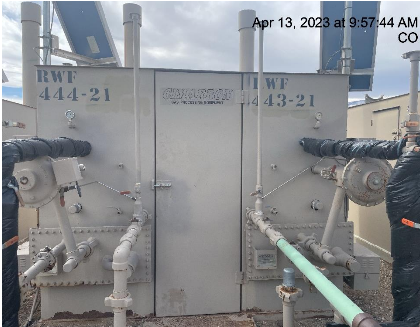
Photo # 5348 Meter calibration info not conspicuously posted
