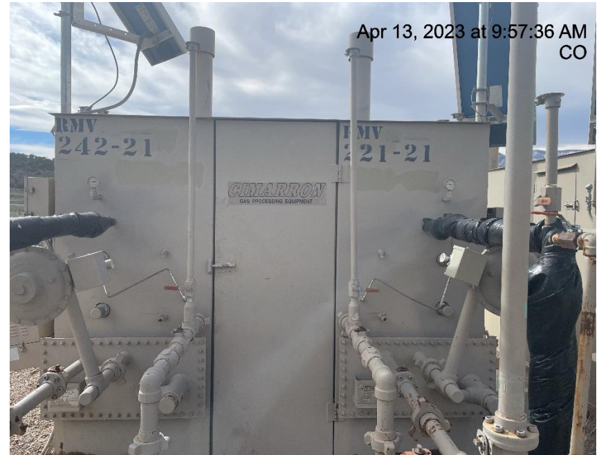
Photo # 5347 Meter calibration info not conspicuously posted
