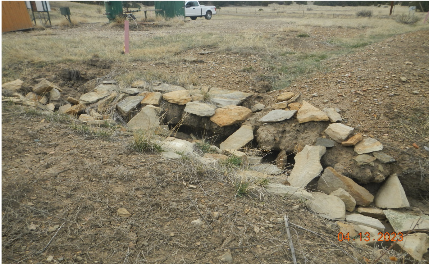
Photo 2. Stormwater is cutting underneath the rip/rap in this area.
