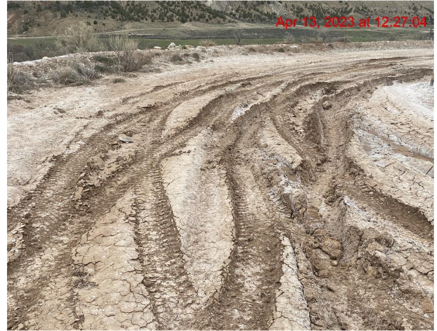
Lack of Stabilization – Photo #02162
