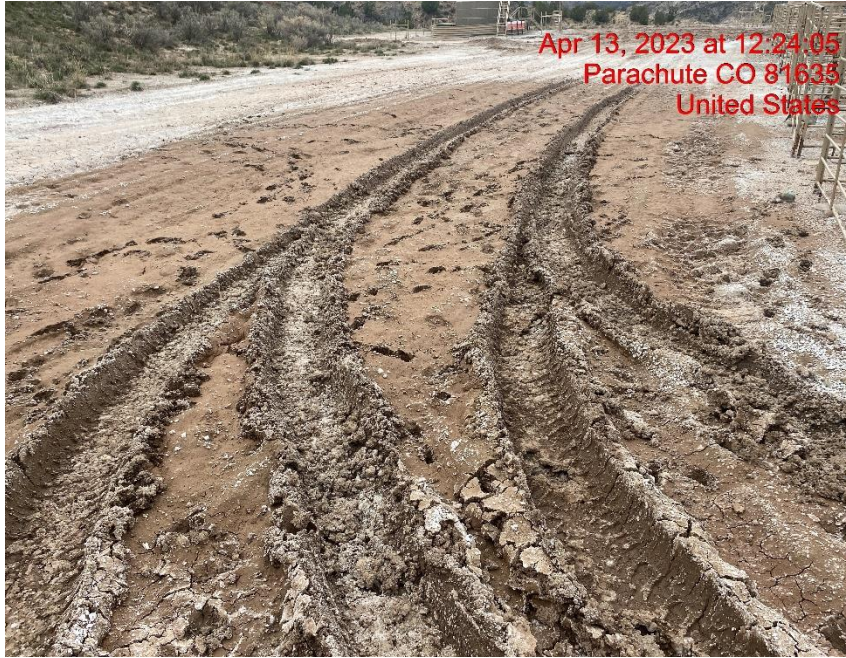
Lack of Stabilization – Photo #02159
