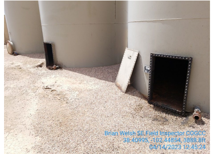
2. East side of oil and water tanks looking at tank hatches. No visible oil noted on the ground and no freestanding fluid was observed
