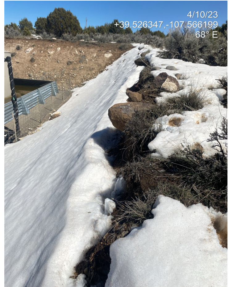
Photo 8. Photos show the cut slope at the south is not stabilized. The lack of stabilization appears to be impacting vegetation areas above and migrating backwards/upslope as is evidenced by eroded/pedestaled vegetation at the top of the slope.
