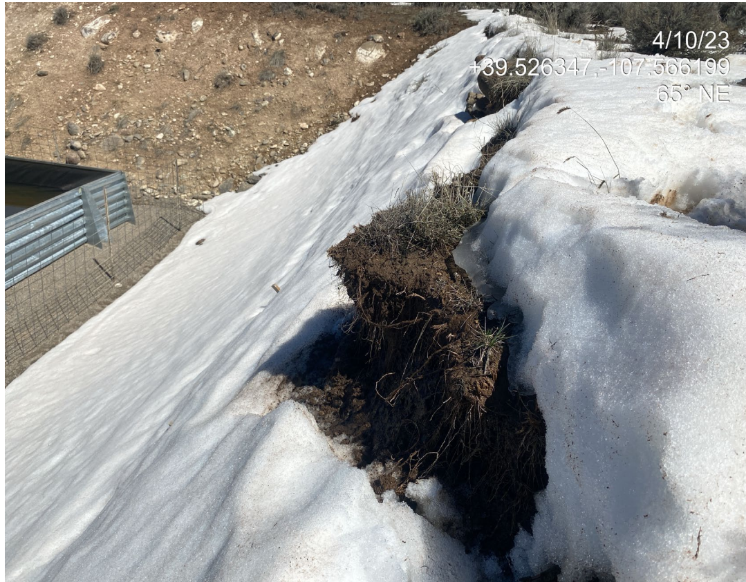
Photo 8. Photos show the cut slope at the south is not stabilized. The lack of stabilization appears to be impacting vegetation areas above and migrating backwards/upslope as is evidenced by eroded/pedestaled vegetation at the top of the slope.
