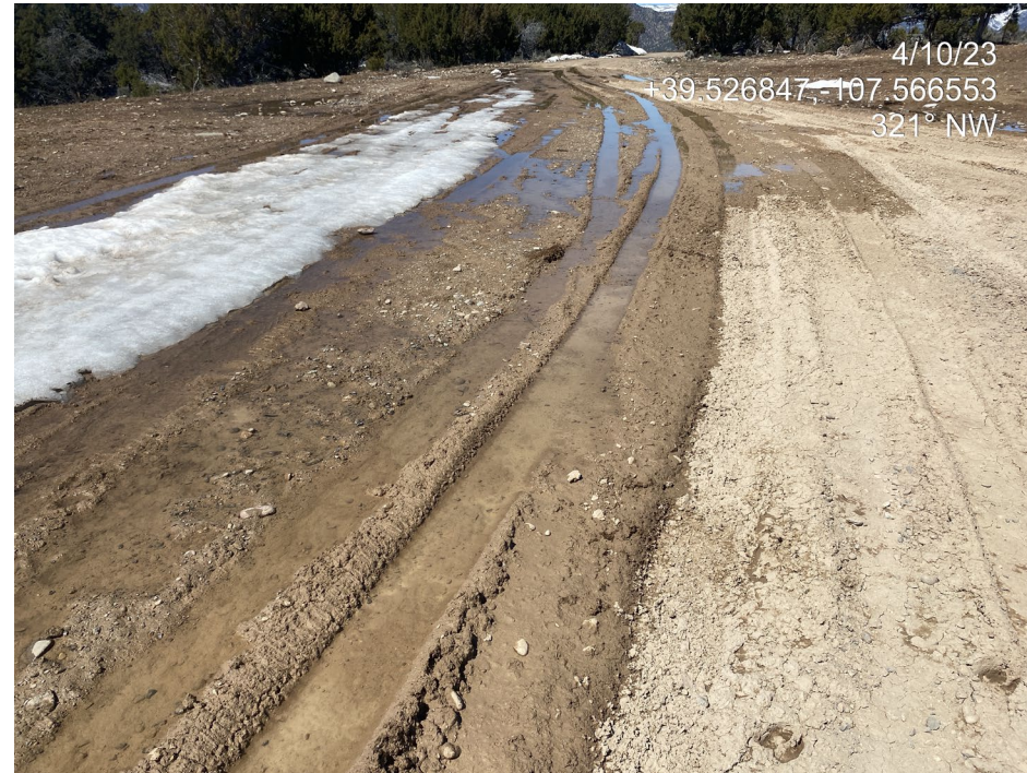
Photo 9. Photos show lack of stabilization of the working pad surface leading towards the access road.
