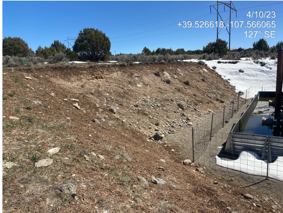
Photo 7. Photos the cut slope at the southeast is not stabilized.
