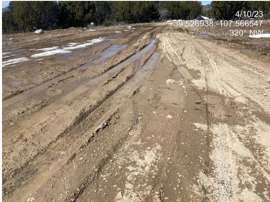
Photo 9. Photos show lack of stabilization of the working pad surface leading towards the access road.
