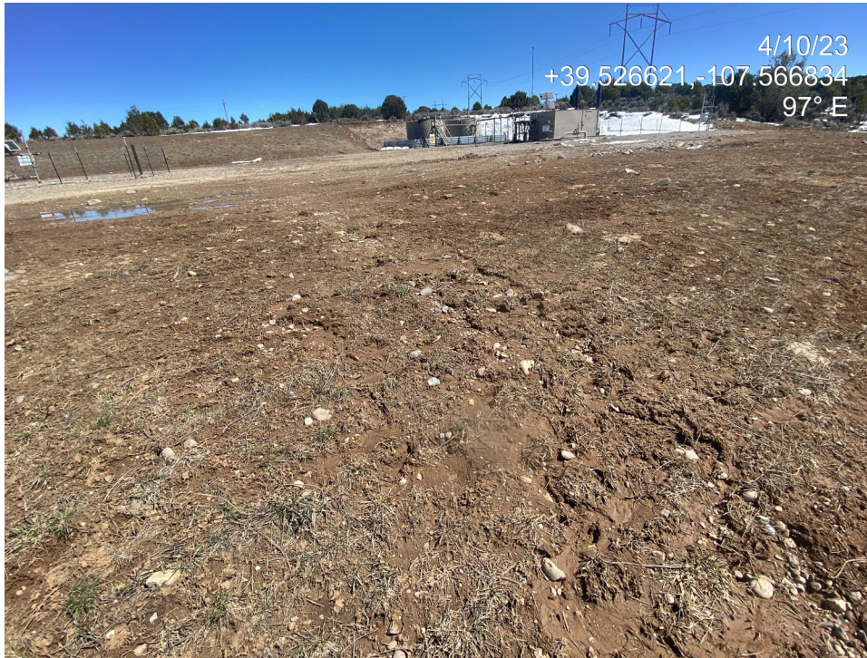
Photo 4. Photos show erosion starting at the western edge of the pad (left) and continuing into the interim area towards a retention pond (right).
