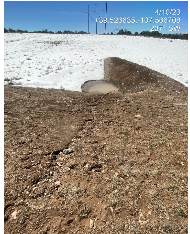
Photo 4. Photos show erosion starting at the western edge of the pad (left) and continuing into the interim area towards a retention pond (right).
