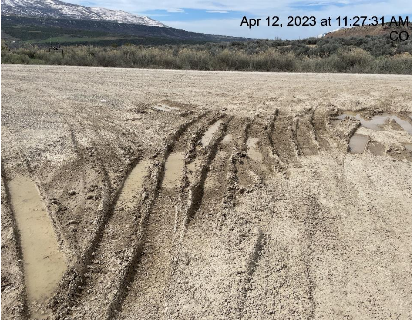
Photo # 5072 Lack of stabilization/compaction
