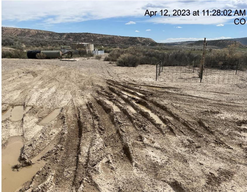
Photo # 5074 Lack of stabilization/compaction
