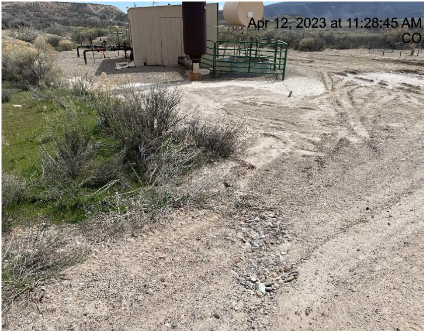
Photo # 5076 Erosion & transport of sediment onto location
