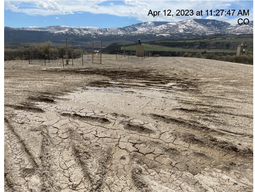
Photo # 5073 Lack of stabilization/compaction
