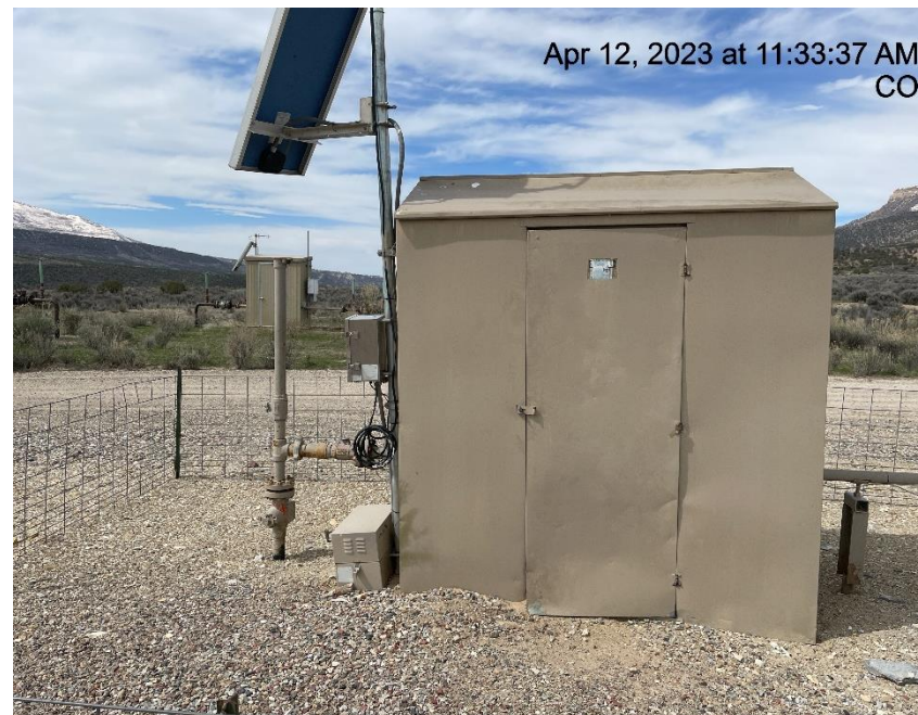
Photo # 5094 Meter calibration info not conspicuously posted
