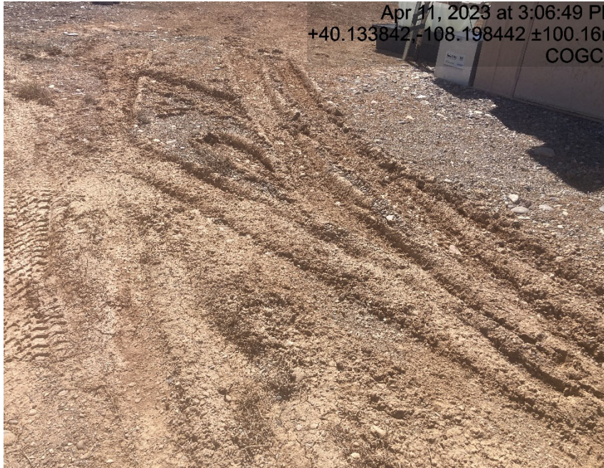
Lack of stabilization/compaction
