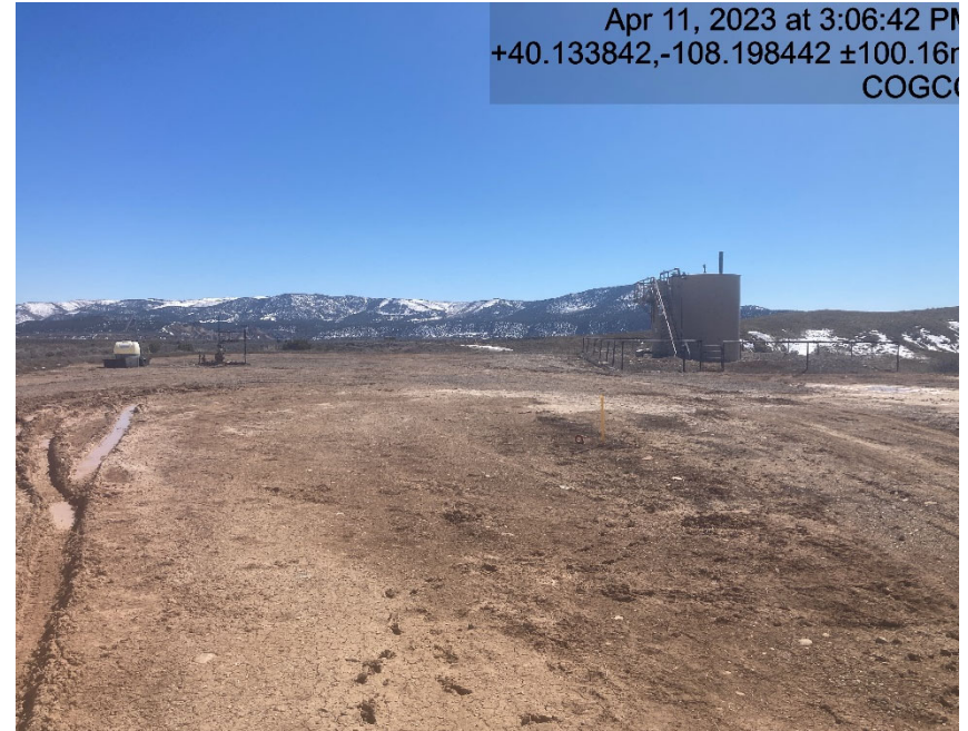
Location and Lack of stabilization/compaction
