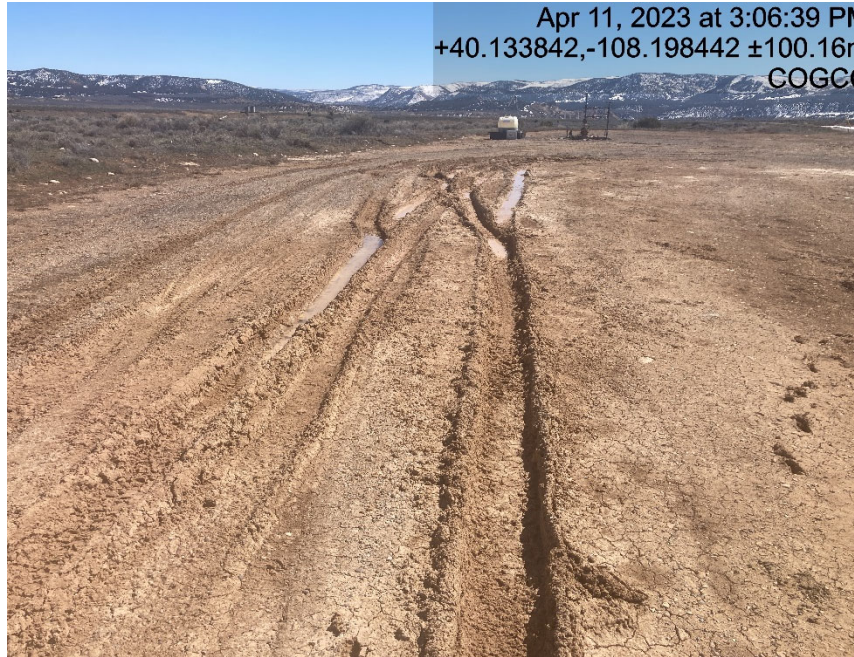
Lack of stabilization/compaction
