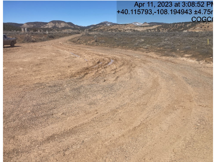
Lack of stabilization/compaction
