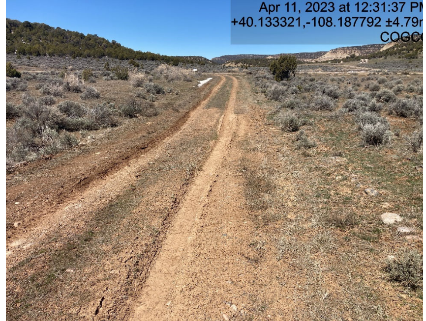
Lack of stabilization on access road and no tracking BMP's
