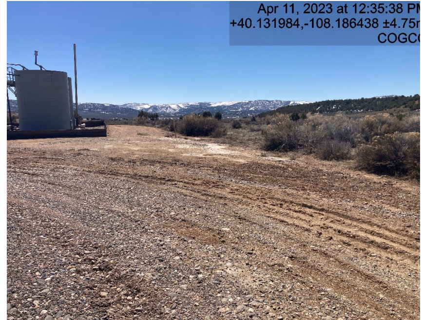
Location lacks BMP's to prevent sediment migration
