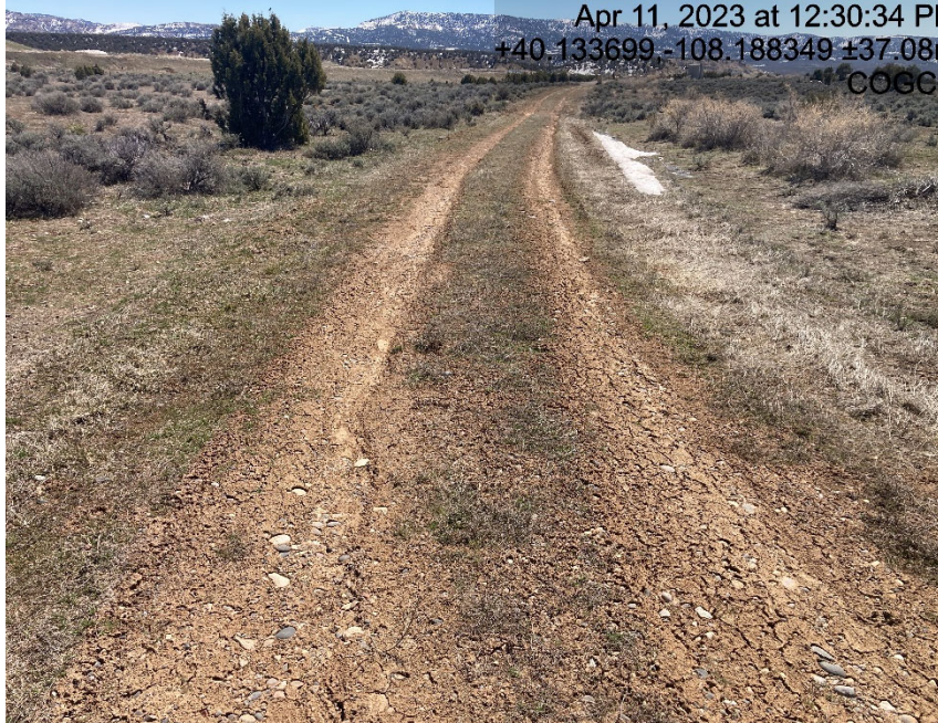
Lack of stabilization on access road and no tracking BMP's
