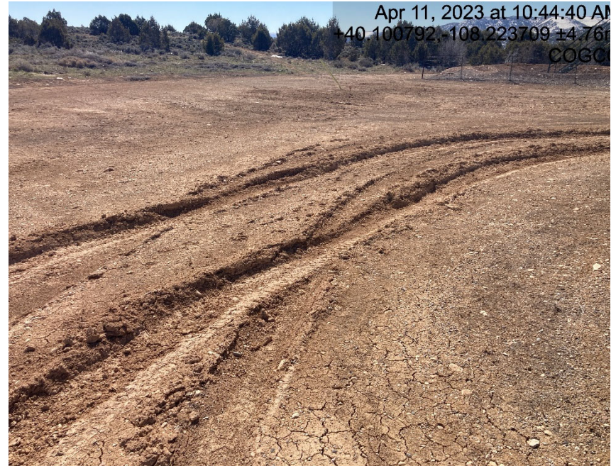
Lack of stabilization/ compaction
