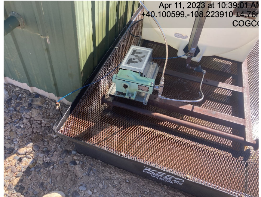
Chemical tank containment is full of fluid
