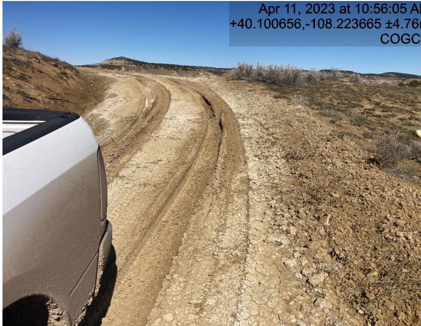
Access road lacks stabilization
