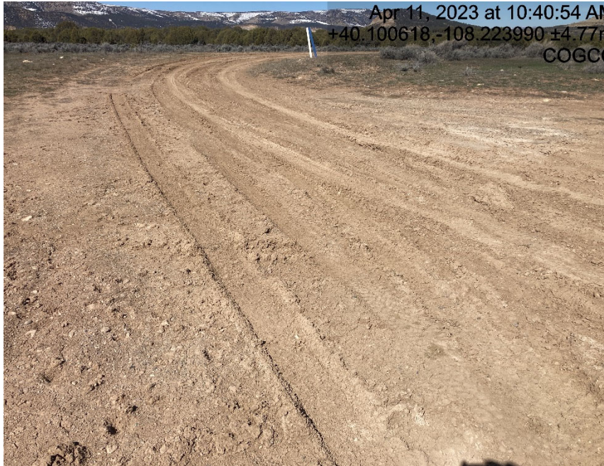
Lack of stabilization/ compaction and no from of tracking BMP's at entrance of location.
