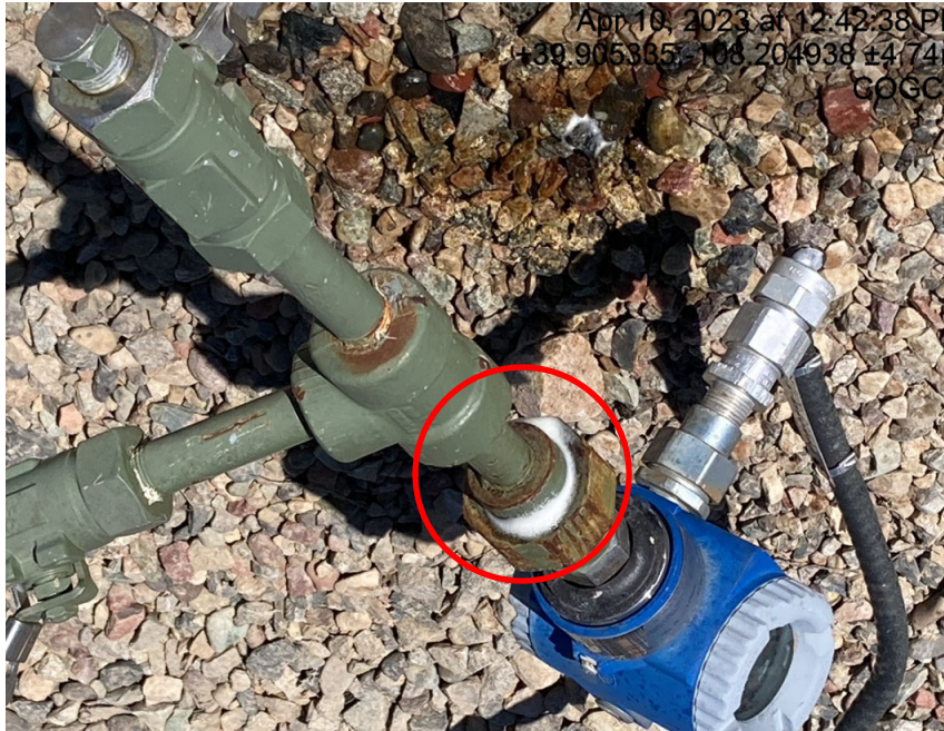
Leaking fitting
