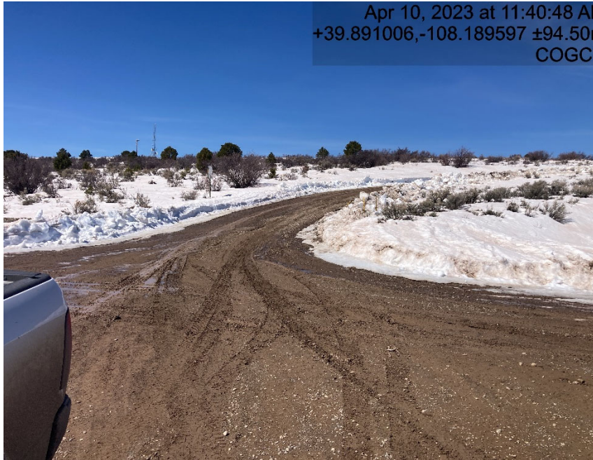
Access entrance to location shows some signs of lack of stabilization
