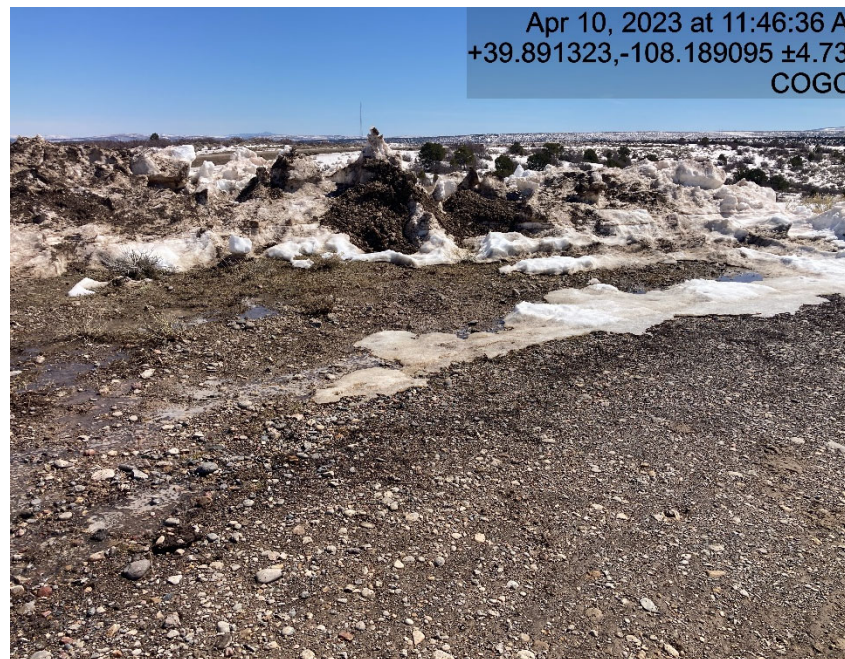
Sediment being pushed off of location
