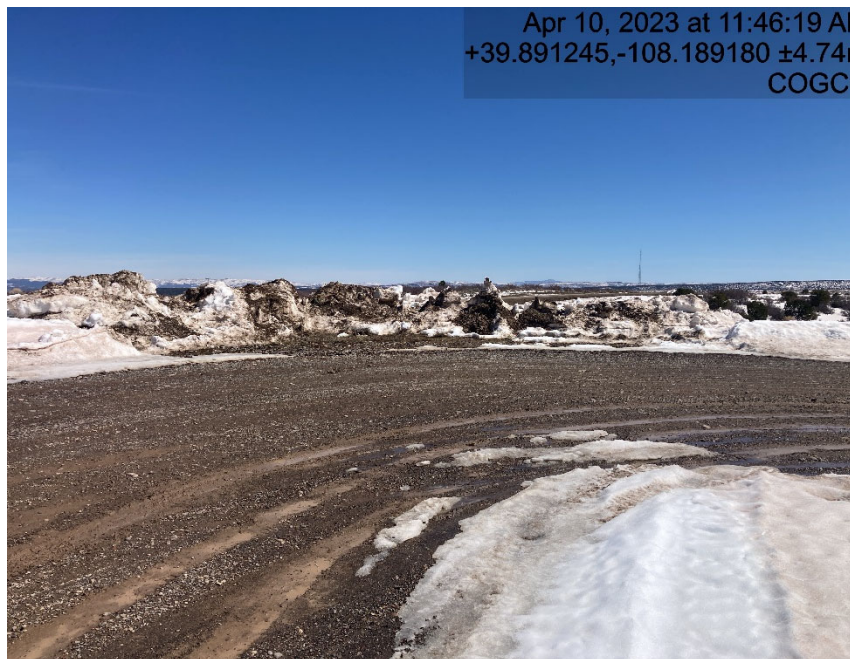
Sediment being pushed off of location
