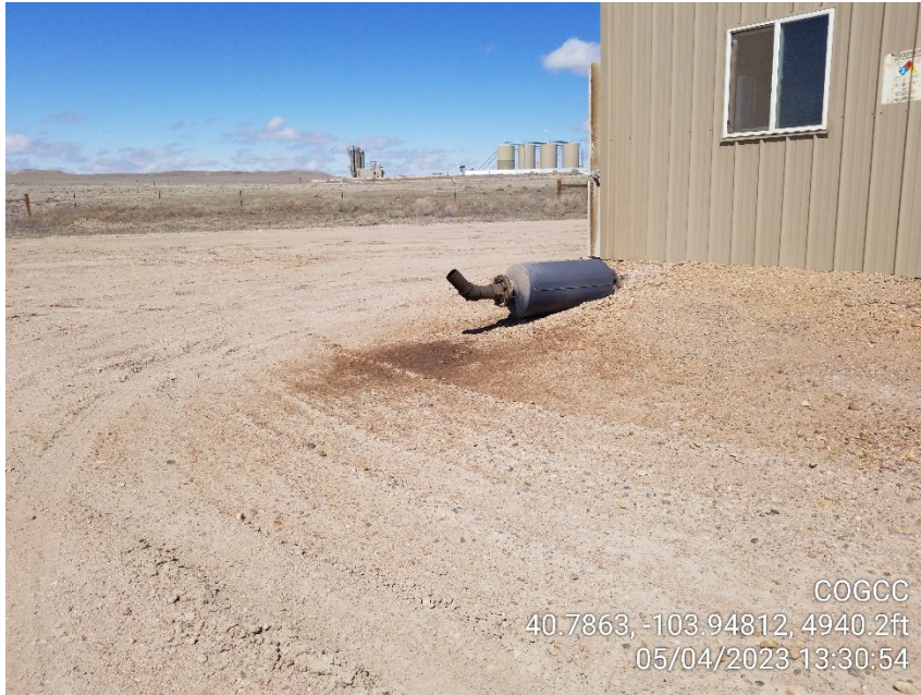
Photo 5 – Stained Soil at Exhaust
