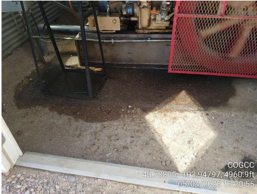
Photo 11 – Gas Engine – Stained Soil
