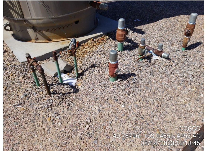
Photo 6 – Unmarked Risers
