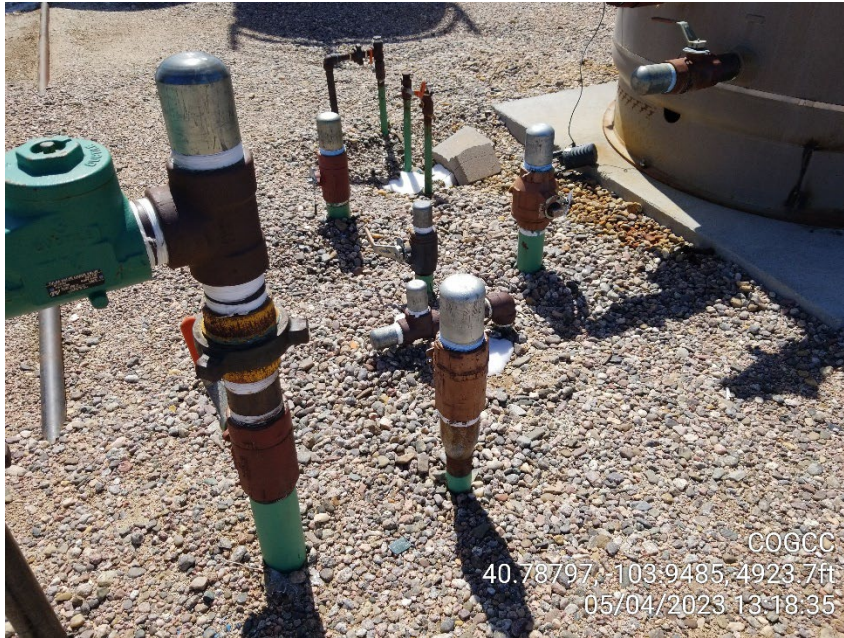
Photo 5 – Unmarked Risers
