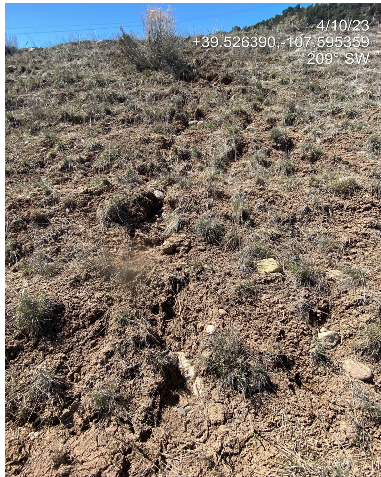
Photo 6. Photos shows where stormwater from the eastern ditch is breaking through the berm (left) and causing degradation to interim areas below (right).
