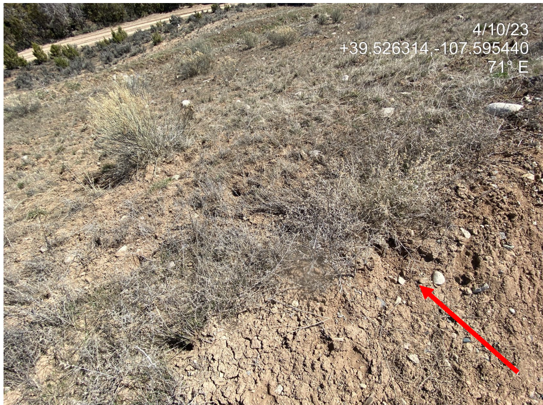
Photo 6. Photos shows where stormwater from the eastern ditch is breaking through the berm (left) and causing degradation to interim areas below (right).
