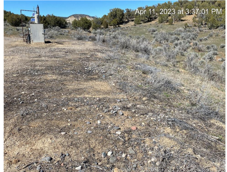
No Stormwater BMP to control sediment migration
