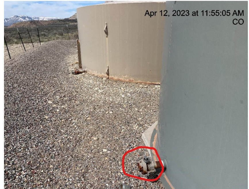
Photo # 5127 Open ended load line
