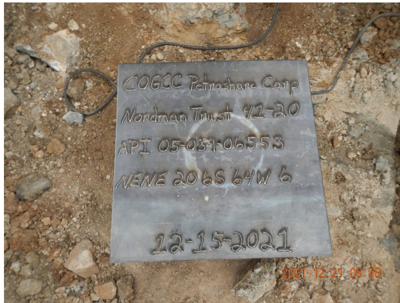
5 – Nordman Trust 41-20 wellhead capped with nameplate
