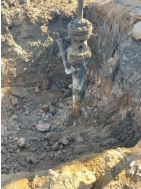
3 – Nordman Trust 41-20 wellhead prior to cut and cap
