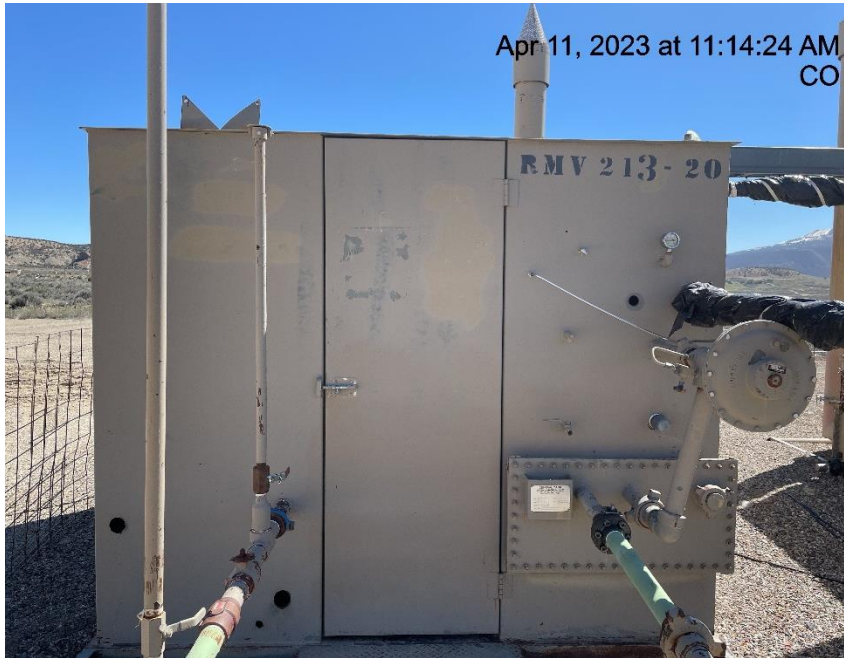
Photo # 5014 Meter calibration info not conspicuously posted
