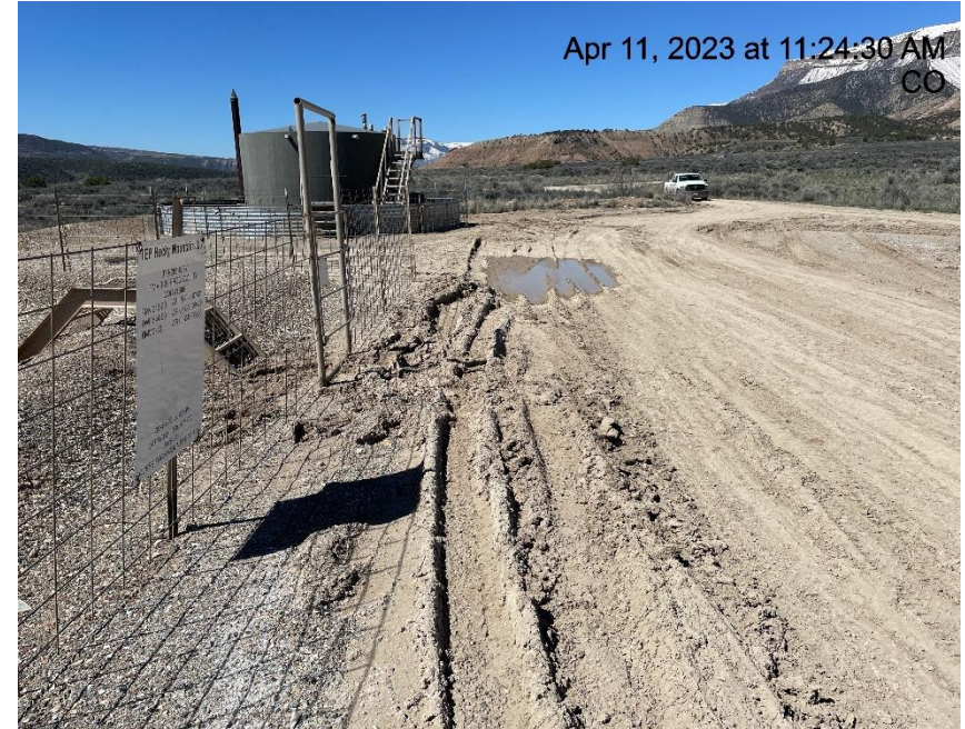
Photo # 5036 Lack of stabilization/compaction
