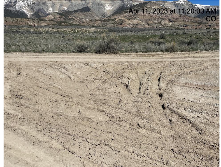
Photo # 5024 Lack of stabilization/compaction
