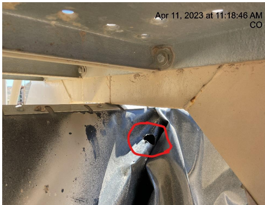
Photo # 5021 Containment liner needs maintenance
