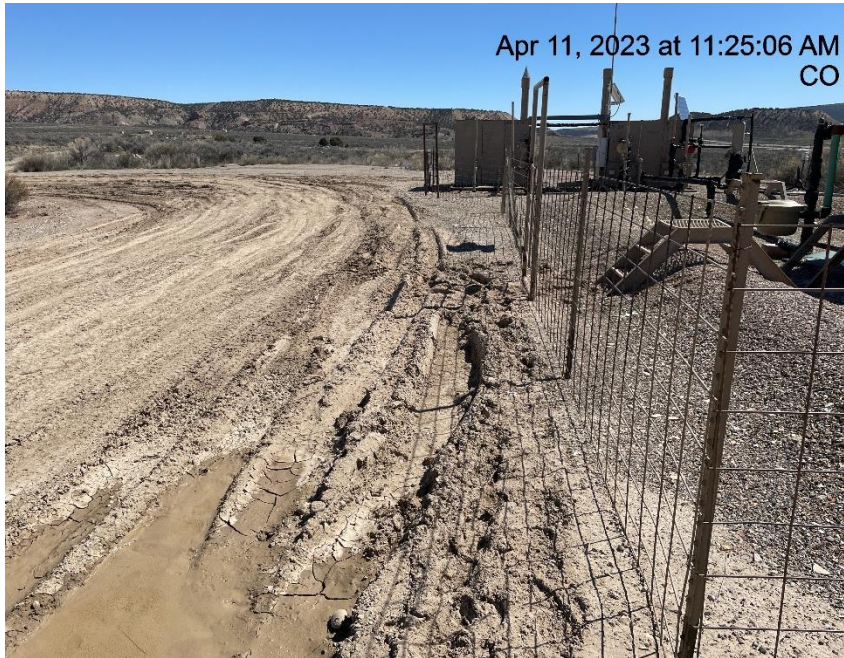
Photo # 5039 Lack of stabilization/compaction
