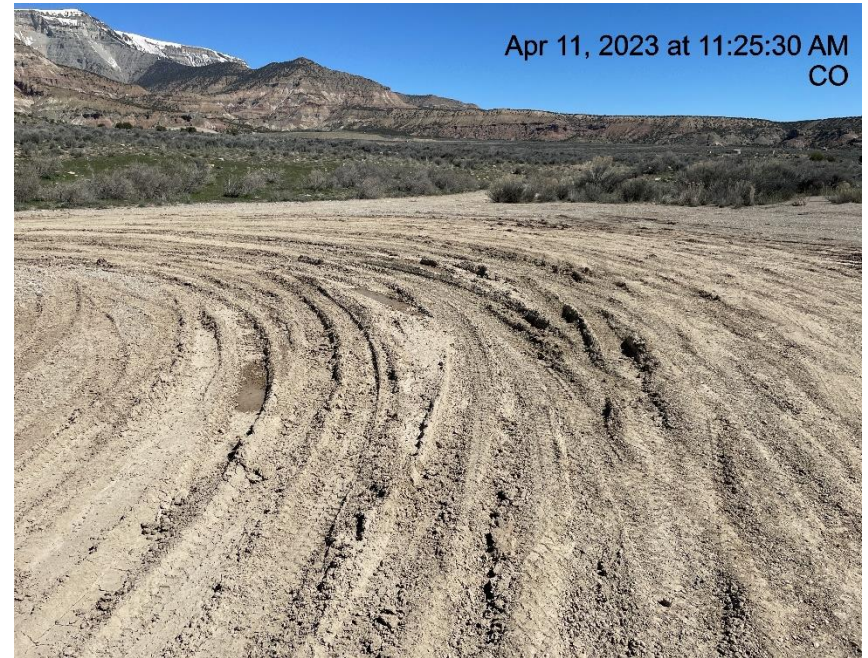
Photo # 5040 Lack of stabilization/compaction
