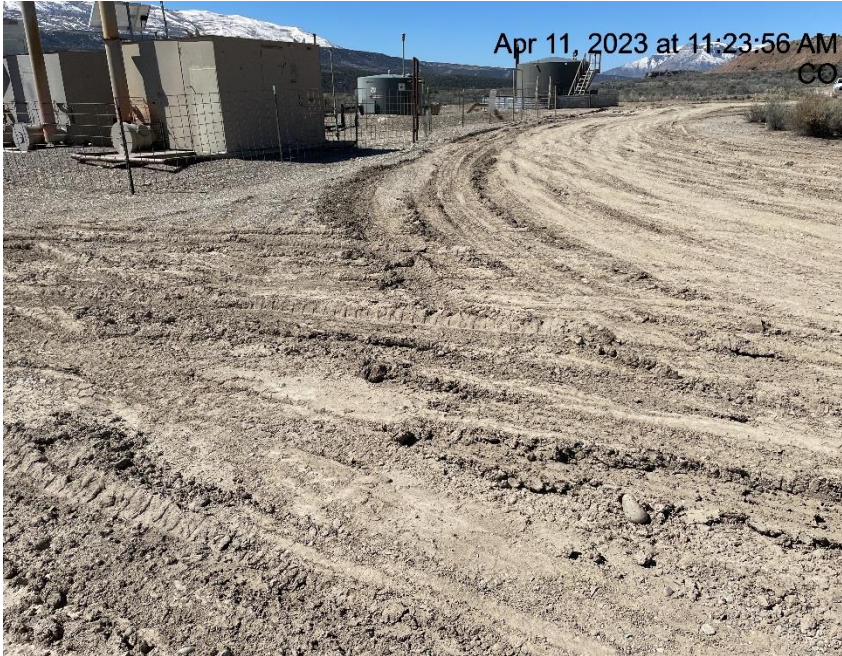
Photo # 5034 Lack of stabilization/compaction
