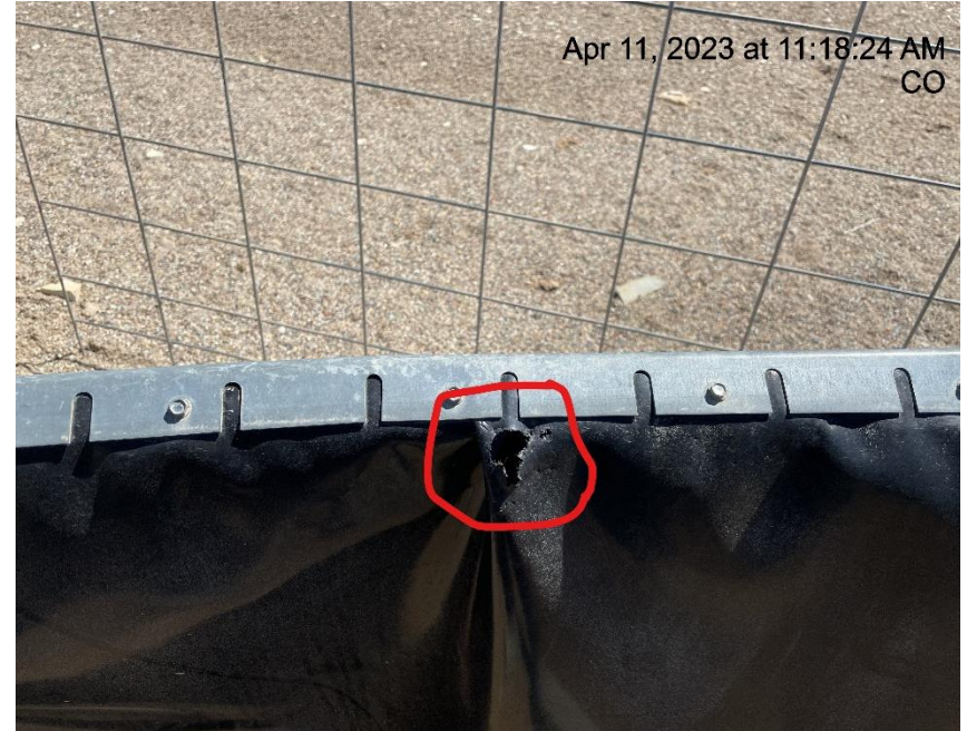
Photo # 5020 Containment liner needs maintenance
