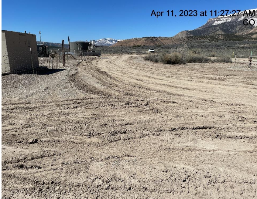
Photo # 5044 Lack of stabilization/compaction
