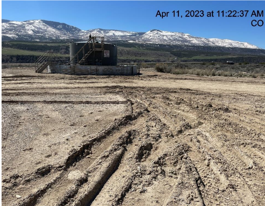
Photo # 5029 Lack of stabilization/compaction
