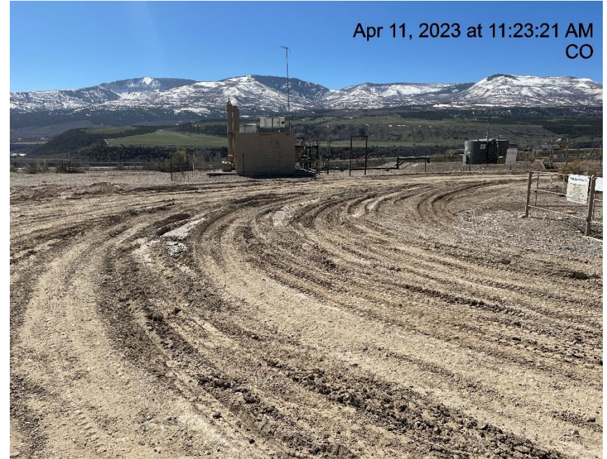
Photo # 5031 Lack of stabilization/compaction
