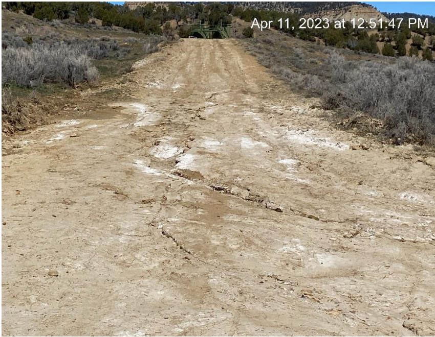
Lease road off county road 143
