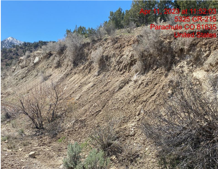
Cut Slope Erosion – Photo #02088
