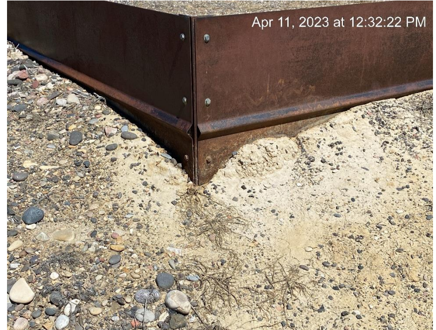
Tank battery containment leak
