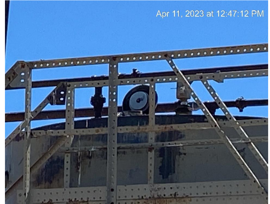
Thief hatch open. Operator sent someone over immediately to close it.
