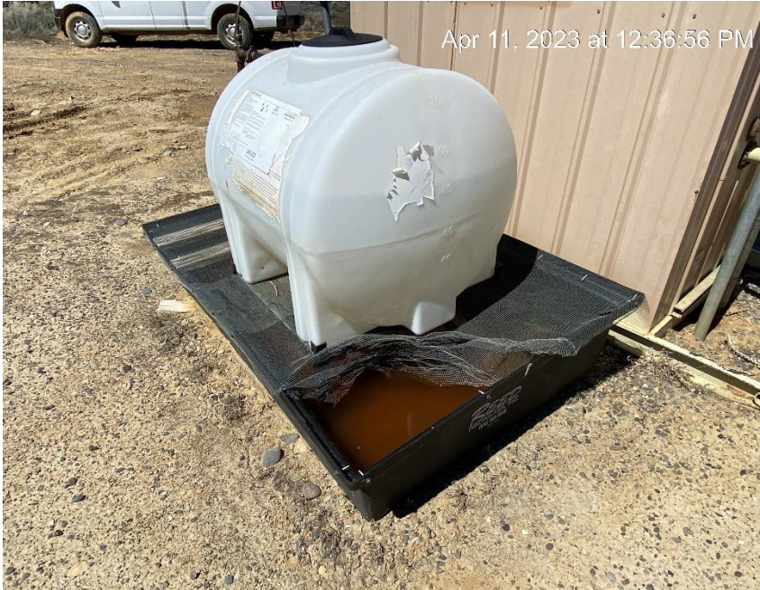
Disconnected, no pump, damaged wildlife netting, containment full of liquid waste
