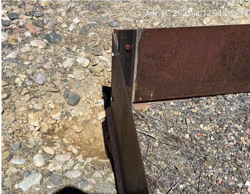
Tank battery containment leak
