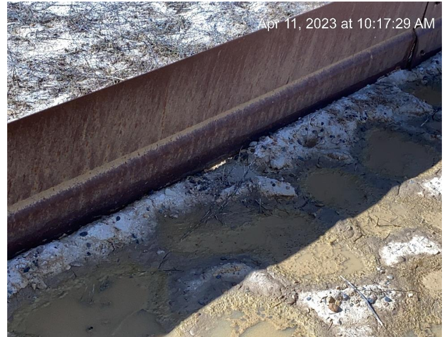
Gap underneath tank containment
