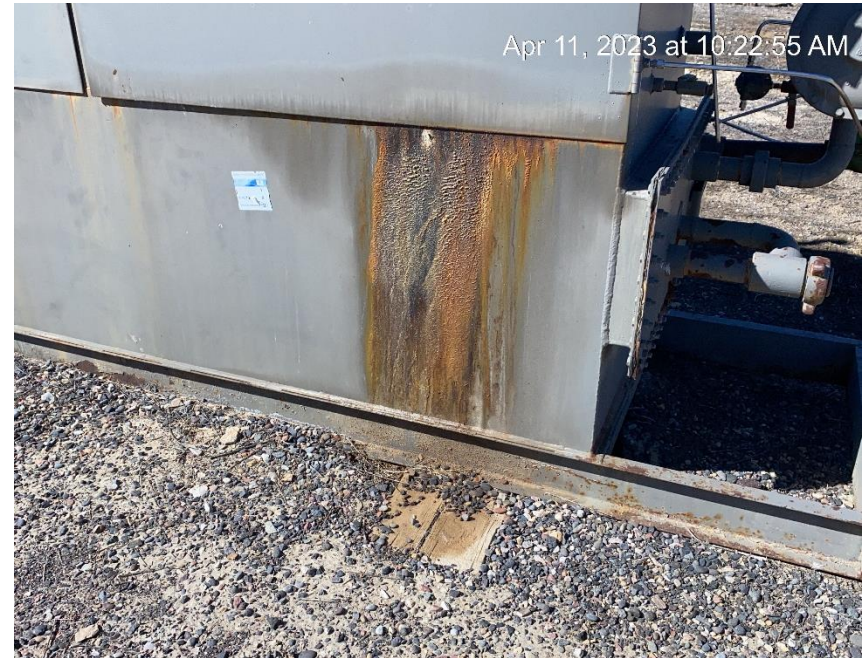
Staining from separator
