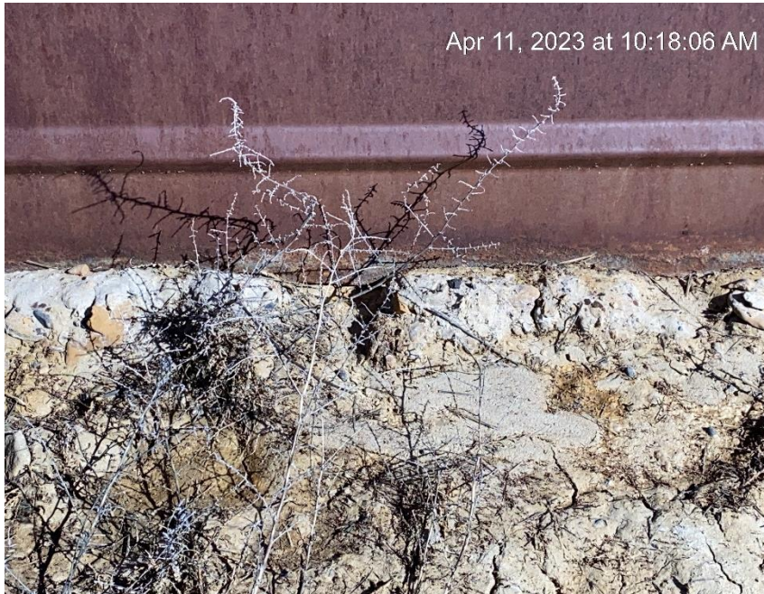
Gap underneath tank containment
