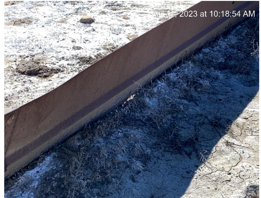
Gap underneath tank containment
