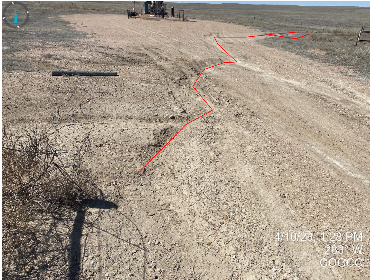
Photo 5. Facing west near the tank battery. Photo illustrates rill erosion occurring on the production areas and exiting off into the interim area. The production area will need to be stabilized and BMPs will need to be installed per good engineering practices to prevent further degradation and sediment transport.
