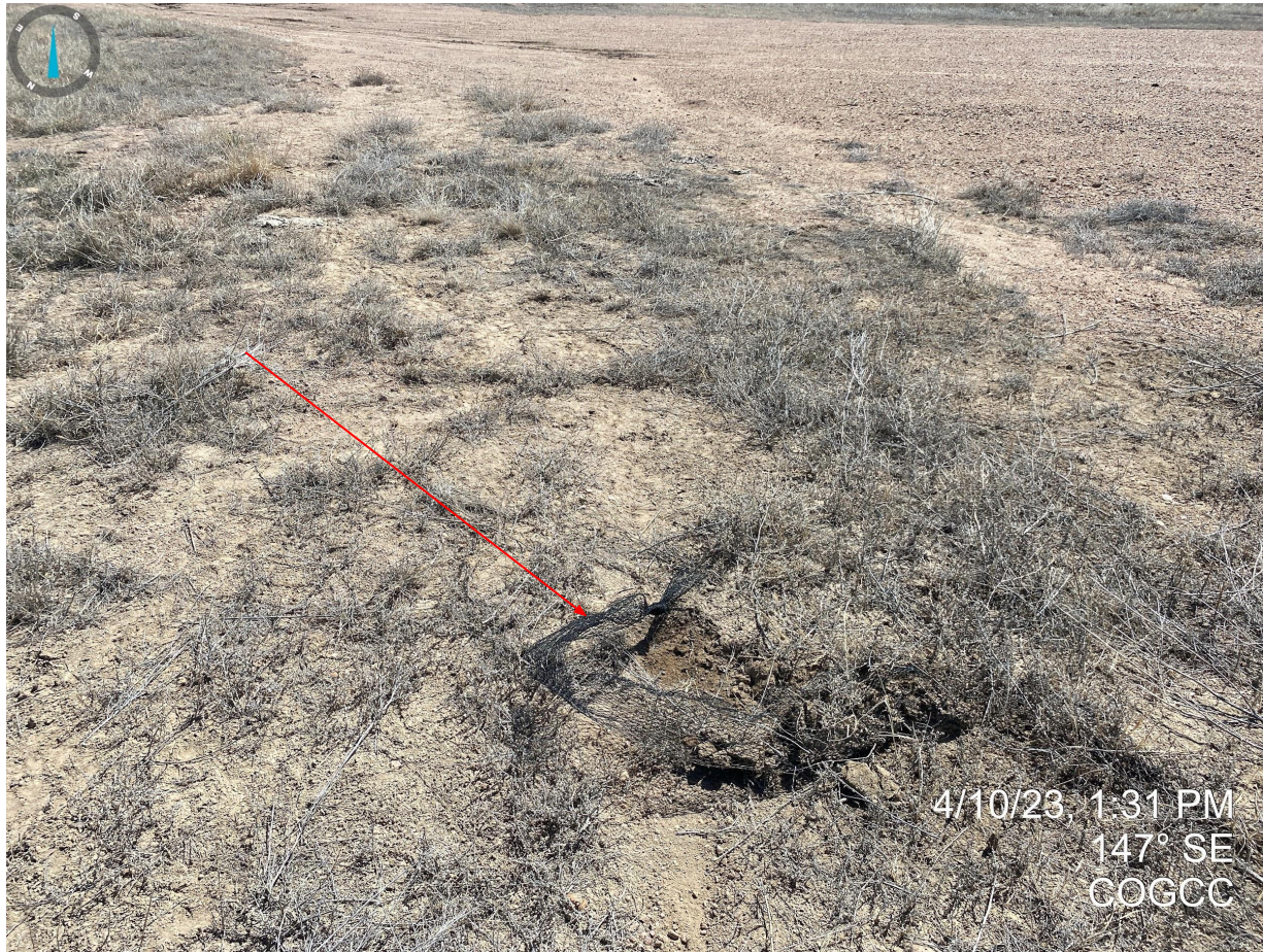
Photo 7. Degraded straw wattle observed on location. This BMP is inadequate and will need to be replaced.
