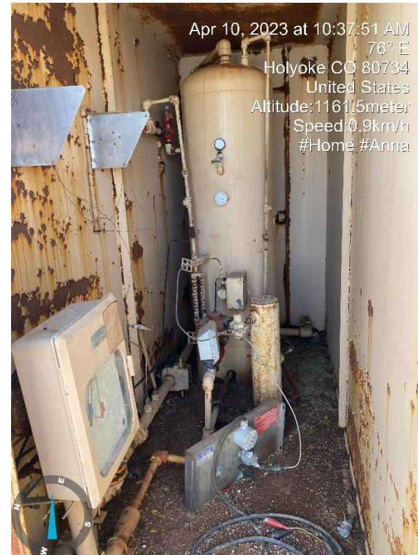
2. Inside Meter shed, Vertical gas separator, gas scrubber, Meter run.
