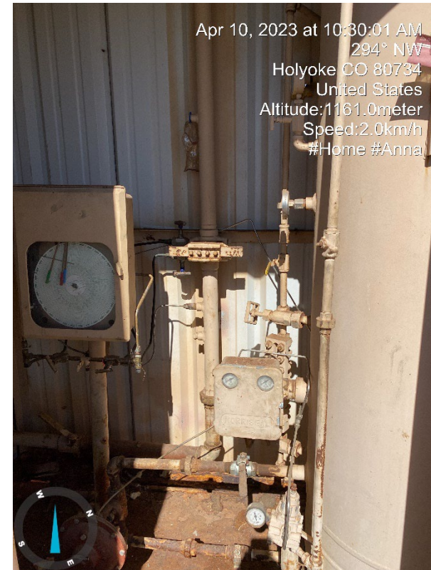
2. Inside Meter shed, Vertical gas separator, Meter run.
