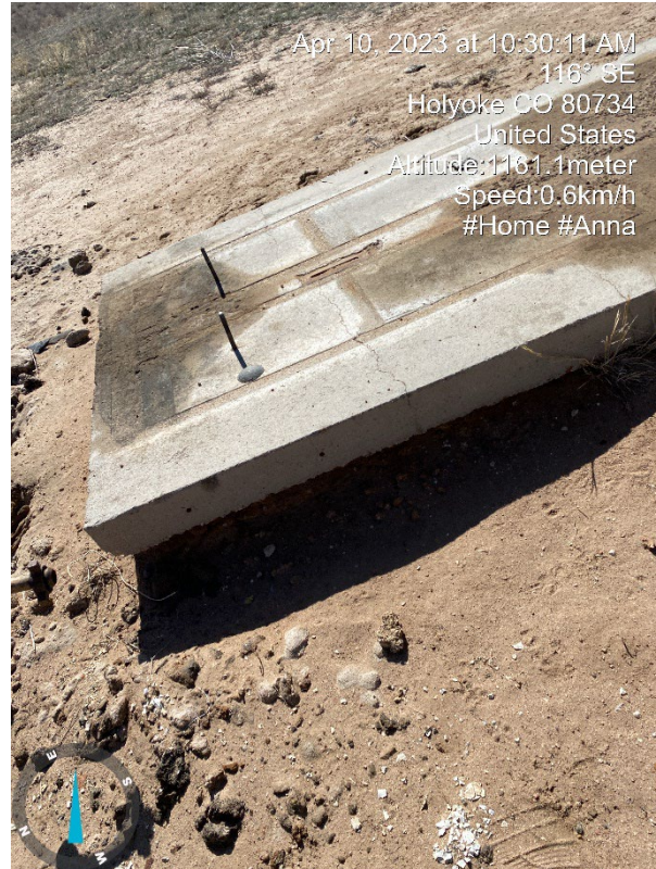
5. Cement pad for pumping unit
