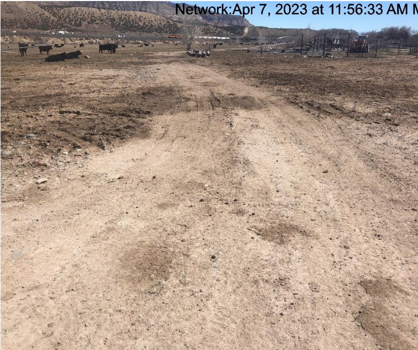
Photo #9601 Insufficient tracking BMP at entrance to location.
