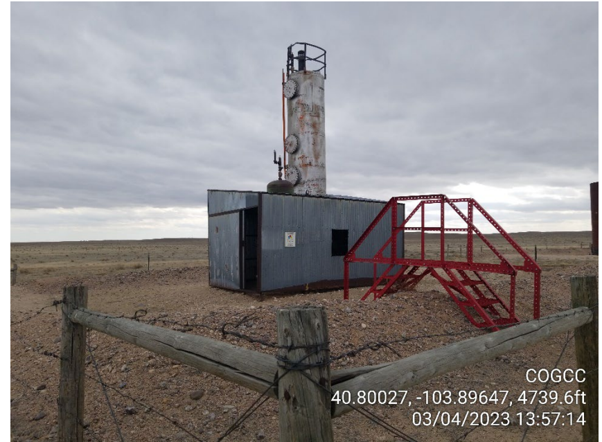
Photo 2 – Heater Treater
