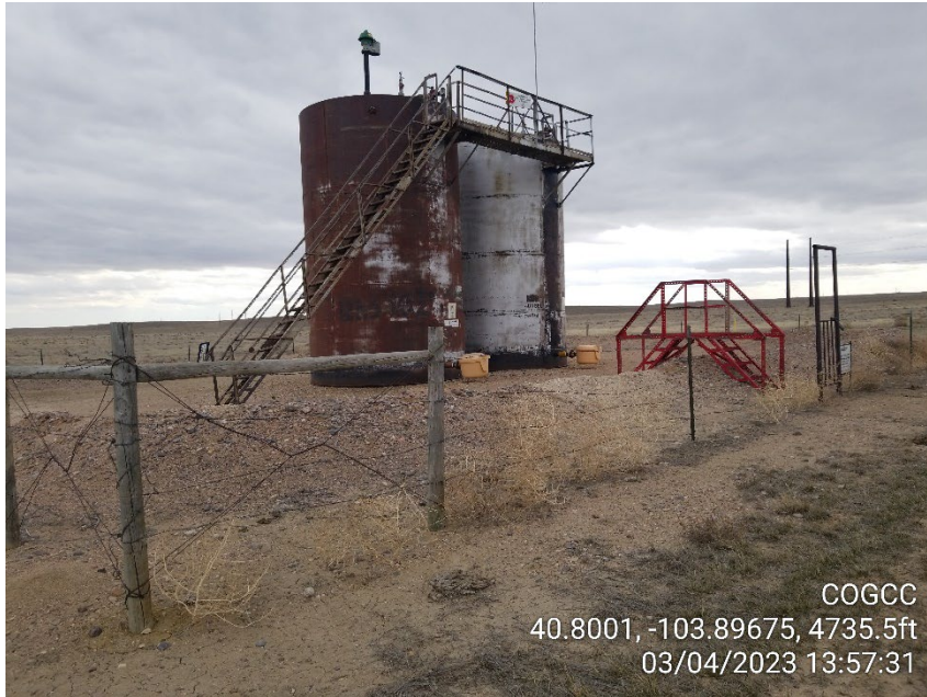
Photo 3 – Tank Battery
