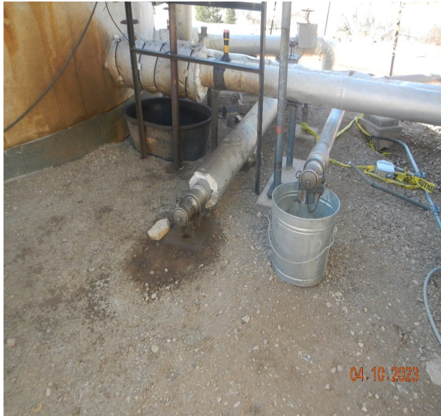
Photo 4. There is oily fluid and stained soil at the pipe outlets of the tank.
