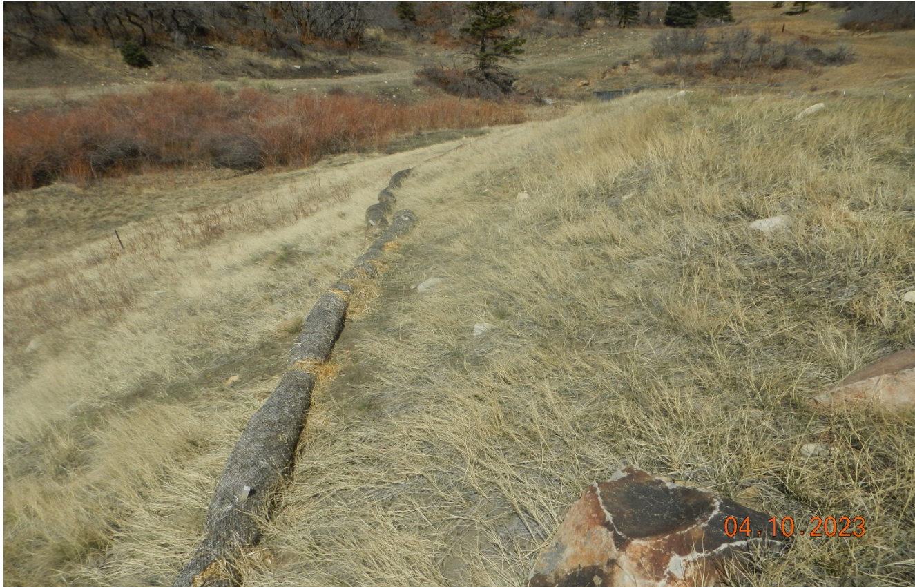
Photo 8. The perimeter wattles are degraded and need to be replaced and maintained.
