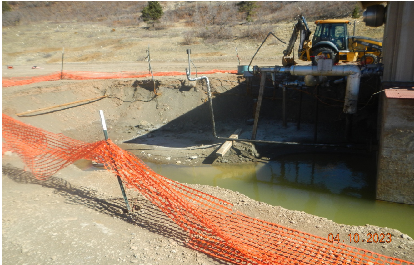
Photo 7. Facing where tank was located which remains an open excavation due to active remediation.
