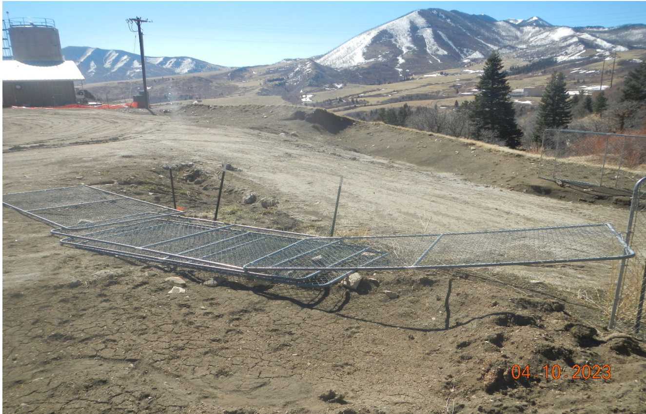
Photo 10. The panels which were around the excavation have fallen over and need to be removed or placed at the other open excavation.
