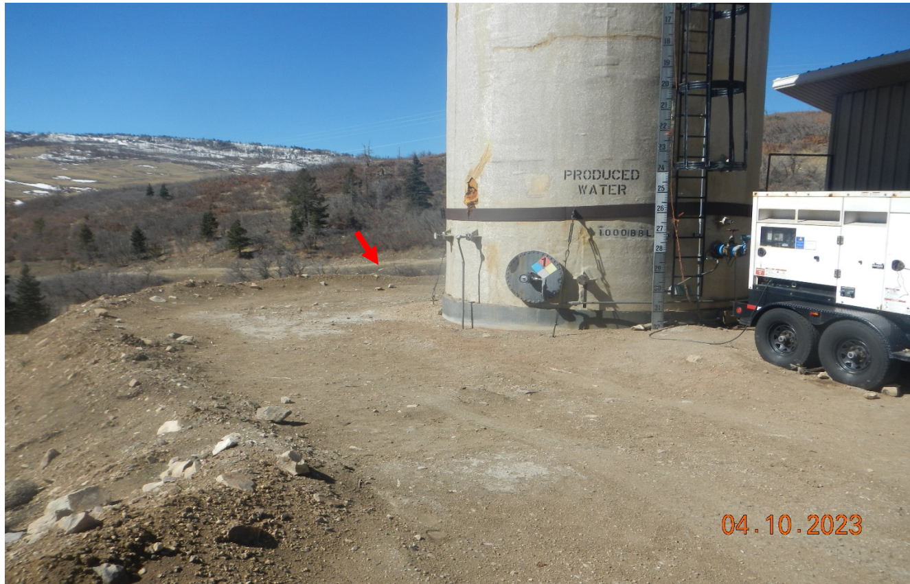
Photo 3. Facing toward the produced water tank. The secondary berm around the tank is insufficient to contain a spill. Red arrow points to small berm which could easily be overtopped by a leak.
