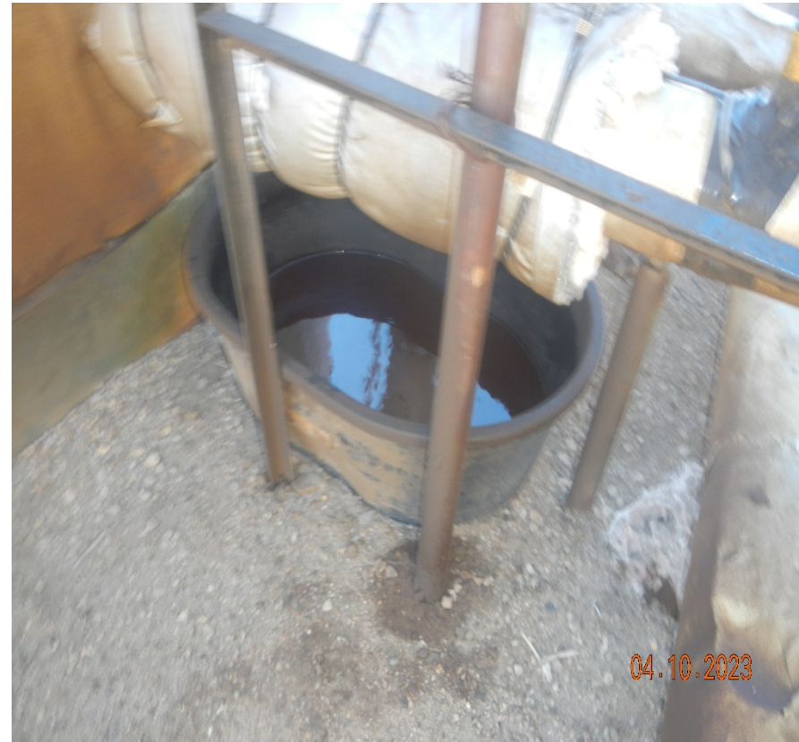
Photo 5. There is oily fluid inside this container used for containment. This needs to be cleaned up and should be netted to prevent wildlife entry.
