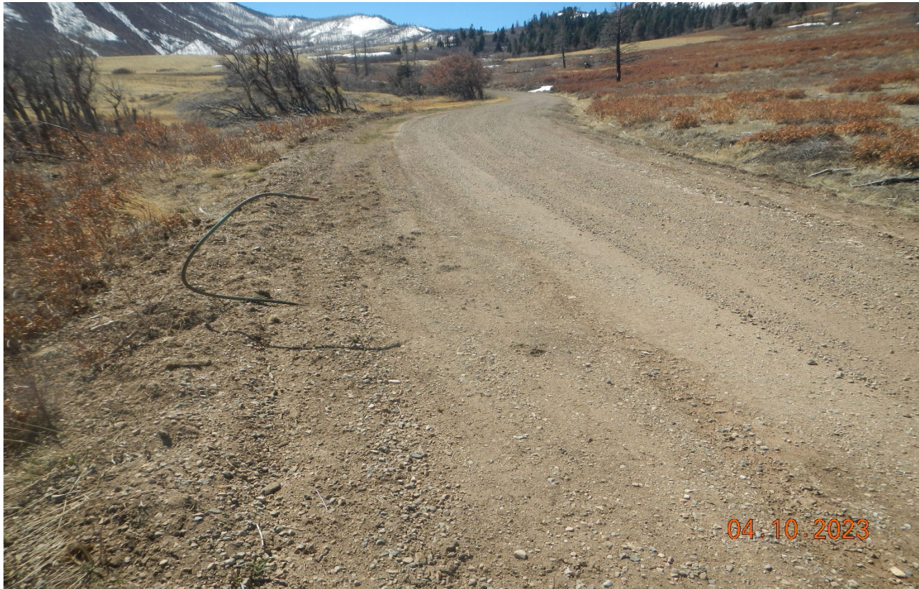
Photo 1. Facing south along the main road. Grading of the road has pushed up the metal rebar and has pushed material and gravel off the roadway. There were a few other bent rebar observed along the road as well.
