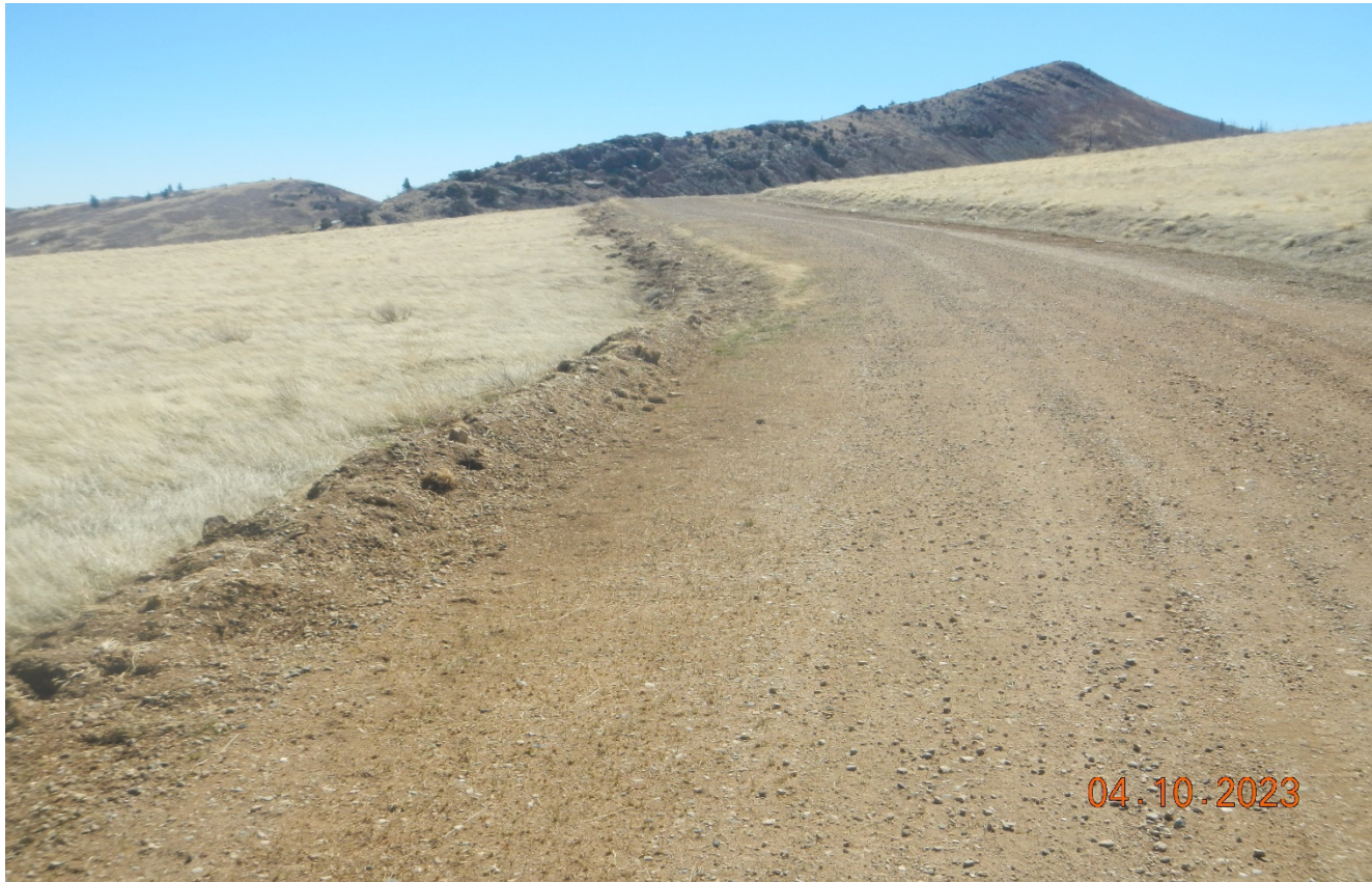
Photo 3. There has been grading performed along the road however, gravel material has been pushed off the road causing additional disturbance This material needs to be removed.
