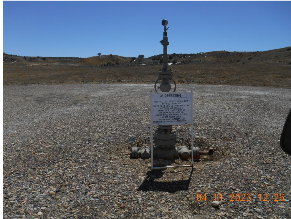
Injection wellhead. Temporarily Abandoned.
