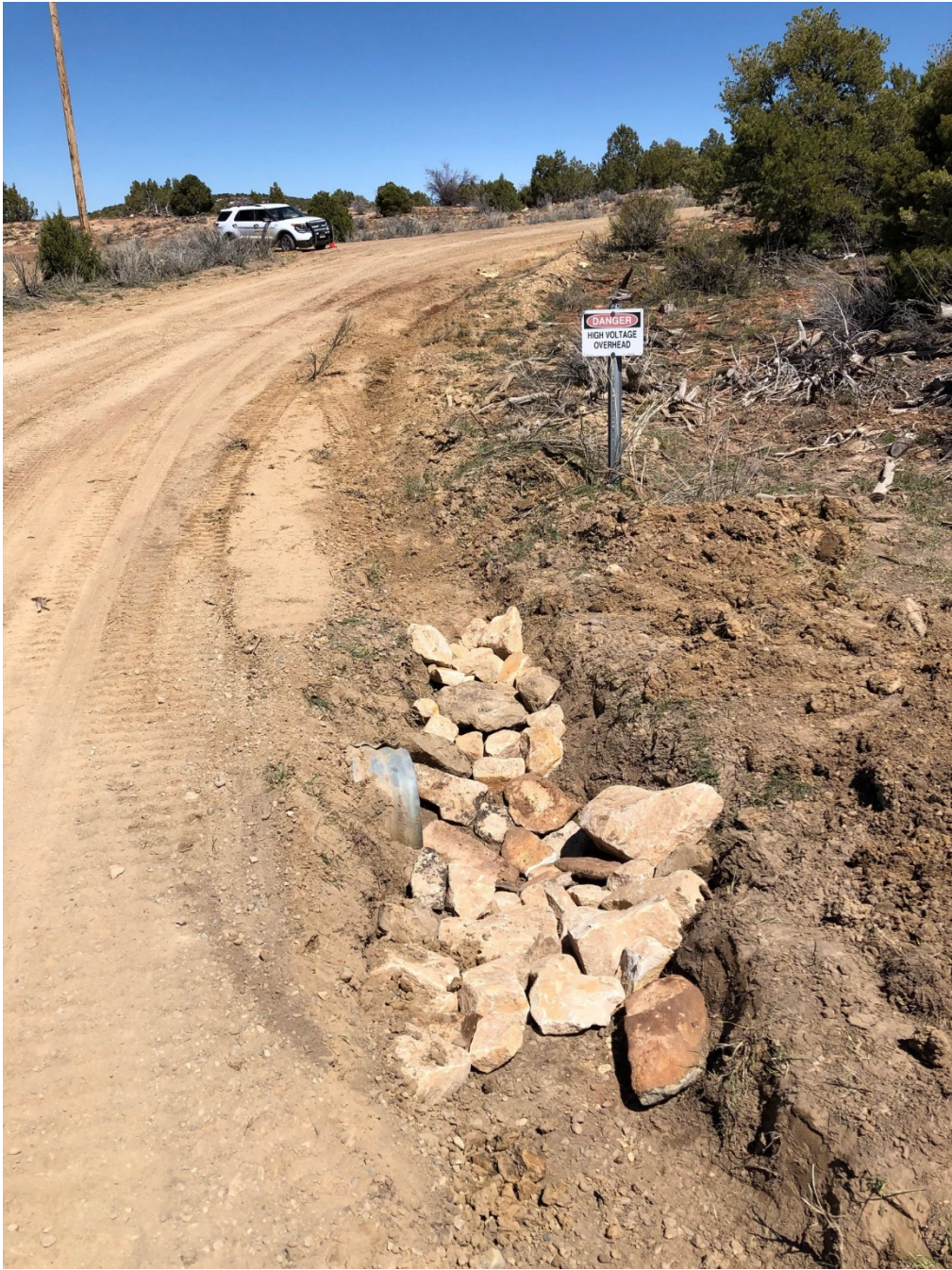
Culvert inlet protected with rock armoring
