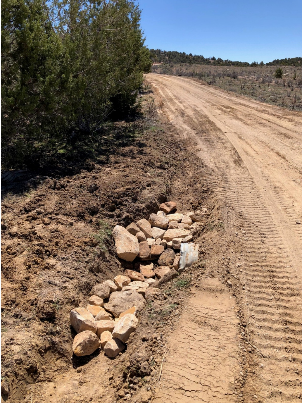
Culvert inlet protected with rock armoring, ditch compacted
