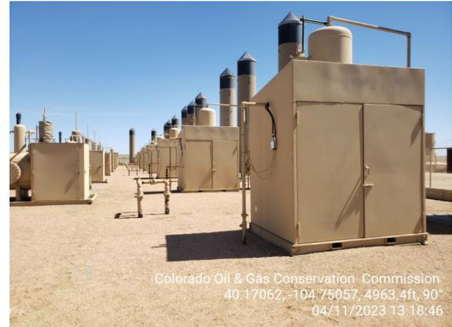
**Photo 7 Horizontal Heated Separators.**
