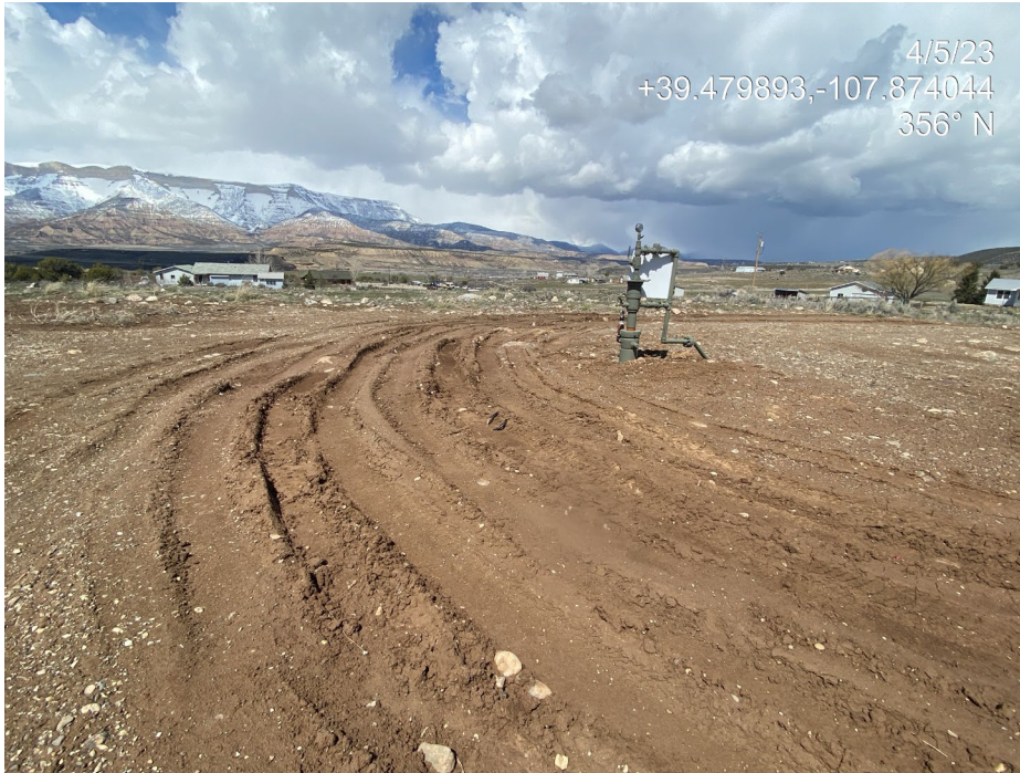
Photo 2. Photos show lack of pad stabilization.
