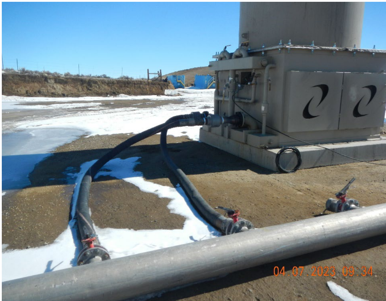
Photo #5 piping to combustor. Valves to the combustor were open from the manifold (at bottom of photo).
