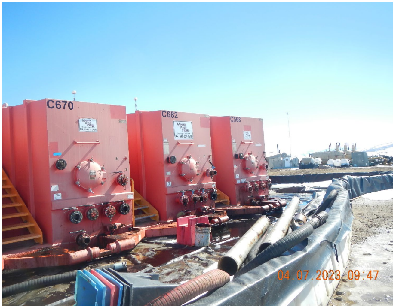
Photo #39 view inside secondary containment of frac tanks.
