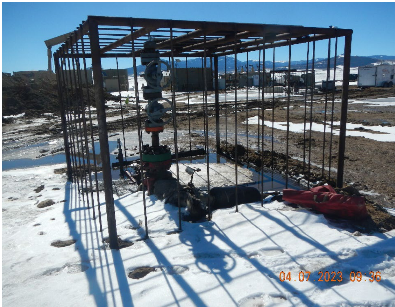
Photo #10 wellhead in cage. Oil on ground around wellhead. Well sign not present. Corrective Action; This area shall be documented on a Remediation workplan (Form 27).
