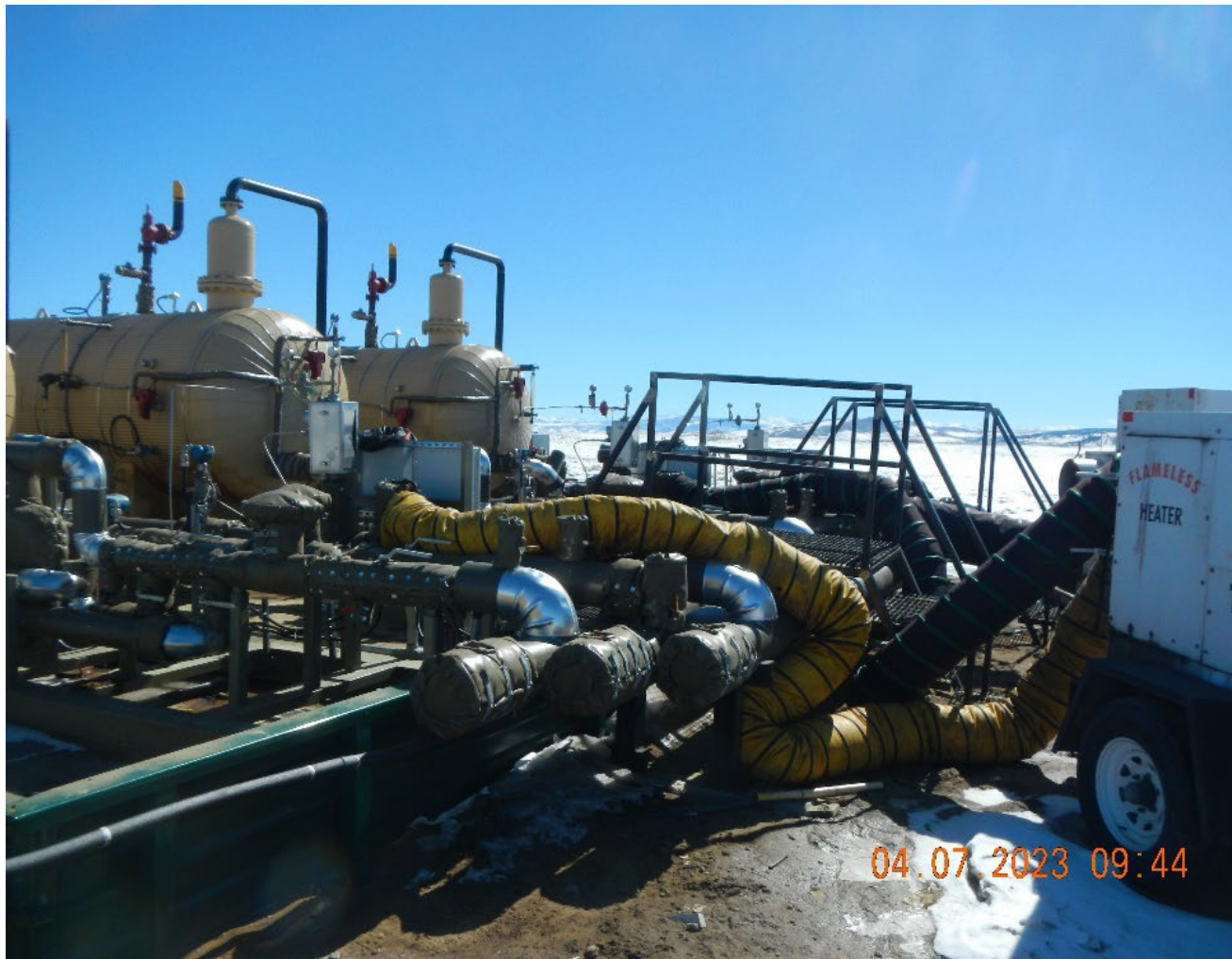
Photo #34 separation equipment with external heaters blowing.
