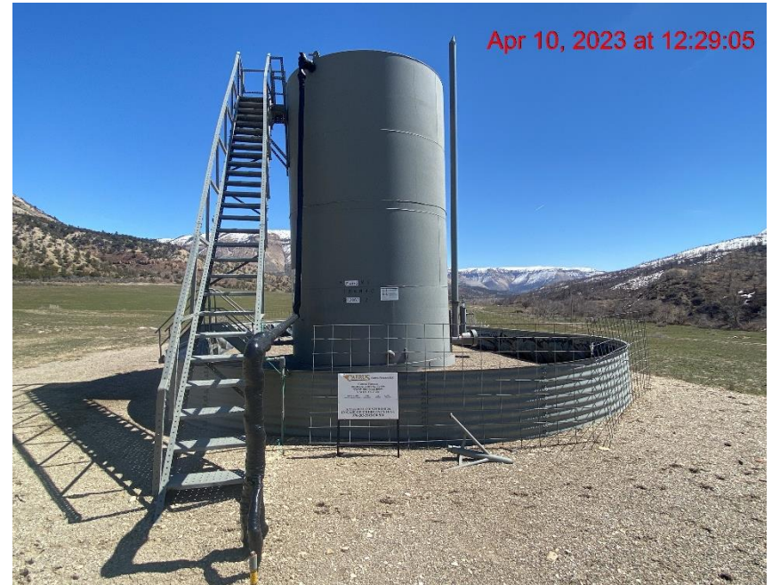
Tank Battery – Photo #02010
