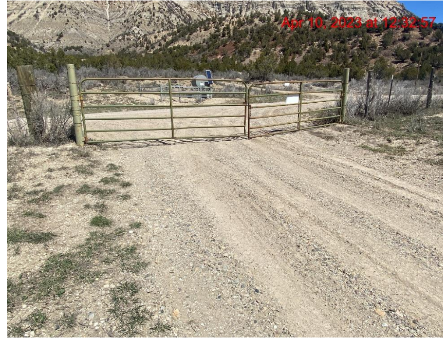
Inadequate Tracking BMP – Photo #02015
