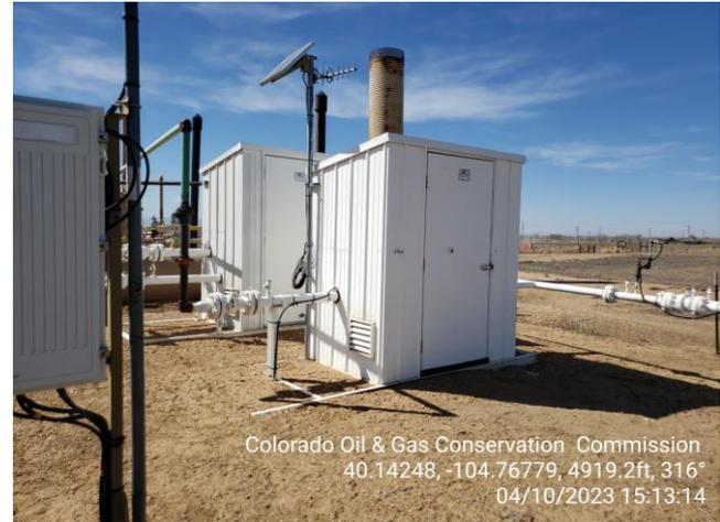
**Photo 5 Horizontal Heated Separators.**
