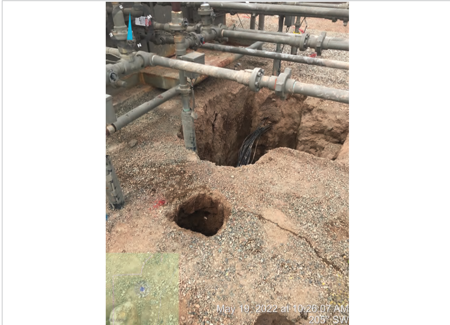
Site Delineation Potholes: View Southwest
