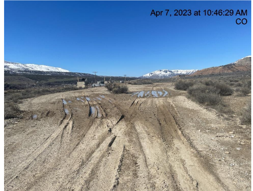
Photo # 4574 Lack of stabilization/Insufficient tracking BMP's
