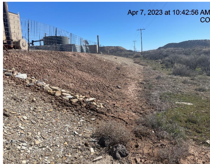
Photo # 4564 Erosion/transport of sediment off location/insufficient BMP's
