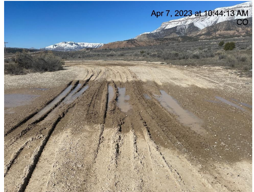
Photo # 4566 Lack of stabilization/compaction/Insufficient tracking BMP's
