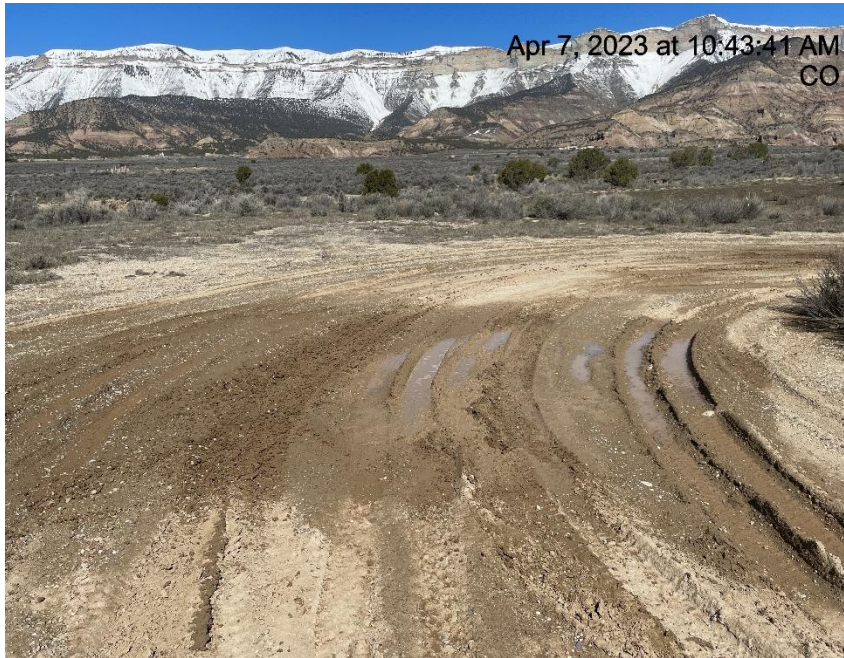
Photo # 4565 Lack of stabilization/compaction/Insufficient tracking BMP's
