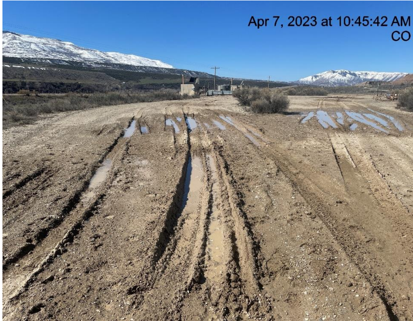
Photo # 4570 Lack of stabilization/Insufficient tracking BMP's
