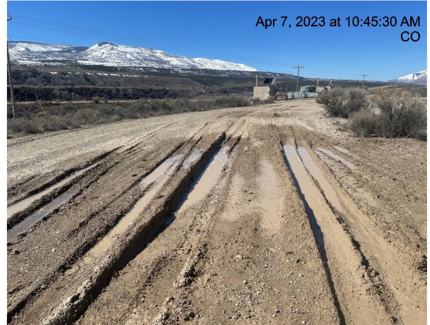
Photo # 4569 Lack of stabilization/compaction/Insufficient tracking BMP's
