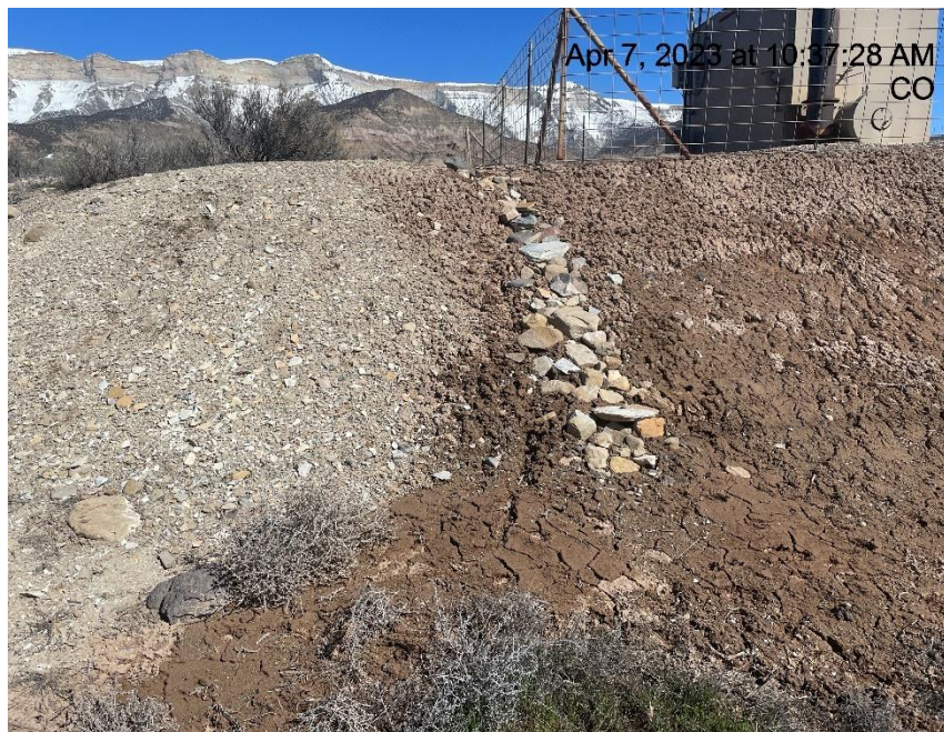
Photo # 4552 Erosion/transport of sediment off location/insufficient BMP's
