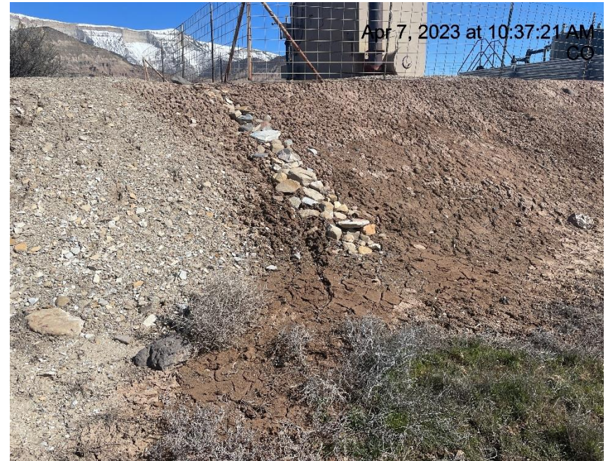
Photo # 4551 Erosion/transport of sediment off location/insufficient BMP's
