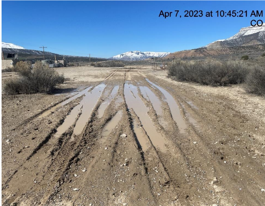
Photo # 4568 Lack of stabilization/compaction/Insufficient tracking BMP's
