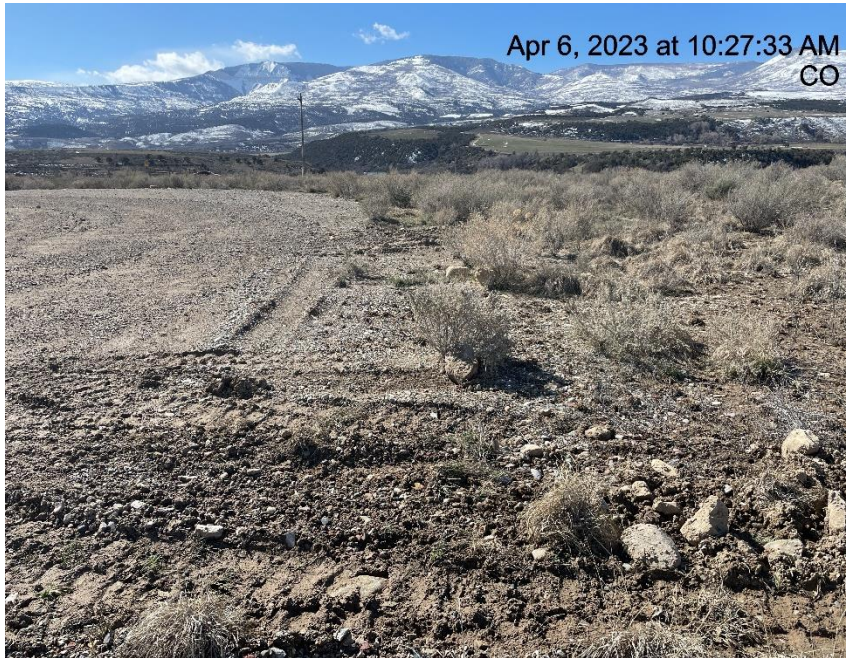
Photo # 4475 Failure to minimize surface disturbance/vehicle tracks into interim area/transport of sediment.
