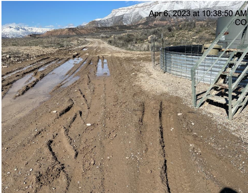
Photo # 4486 Lack of stabilization/insufficient tracking BMP's
