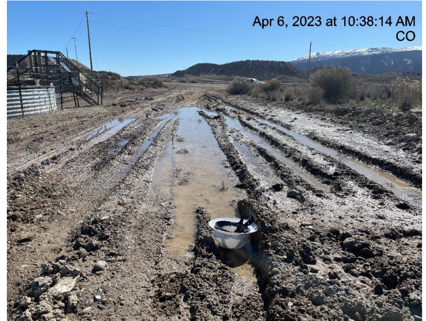
Photo # 4485 Lack of stabilization/insufficient tracking BMP's
