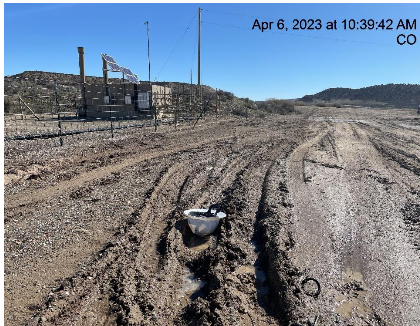
Photo # 4489 Lack of stabilization/insufficient tracking BMP's
