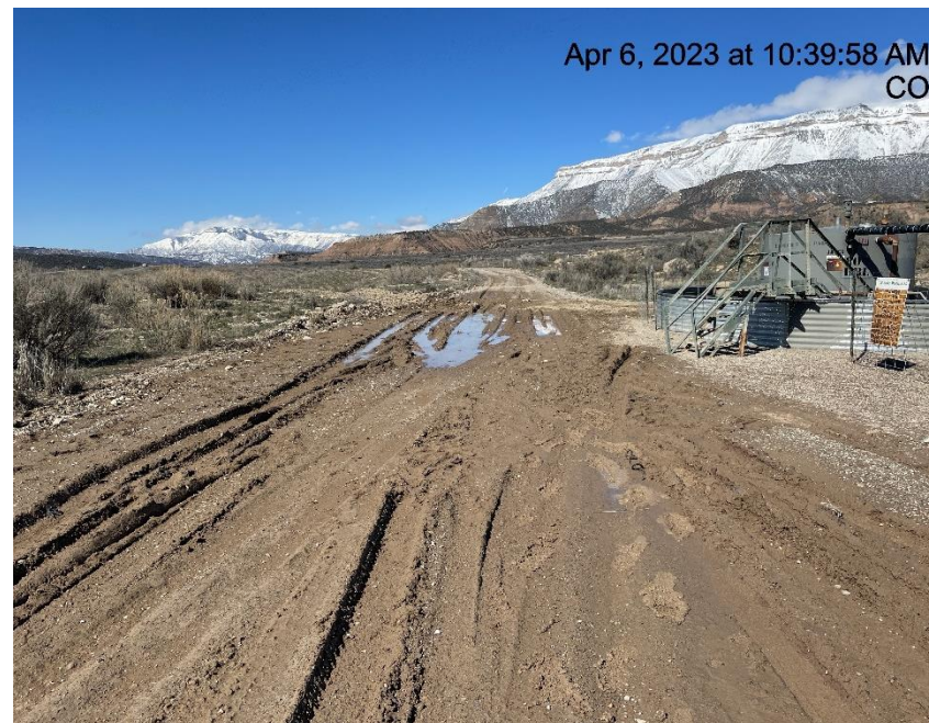
Photo # 4490 Lack of stabilization/insufficient tracking BMP's
