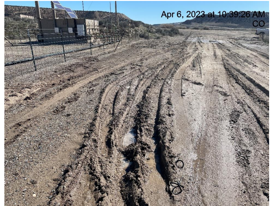
Photo # 4488 Lack of stabilization/insufficient tracking BMP's
