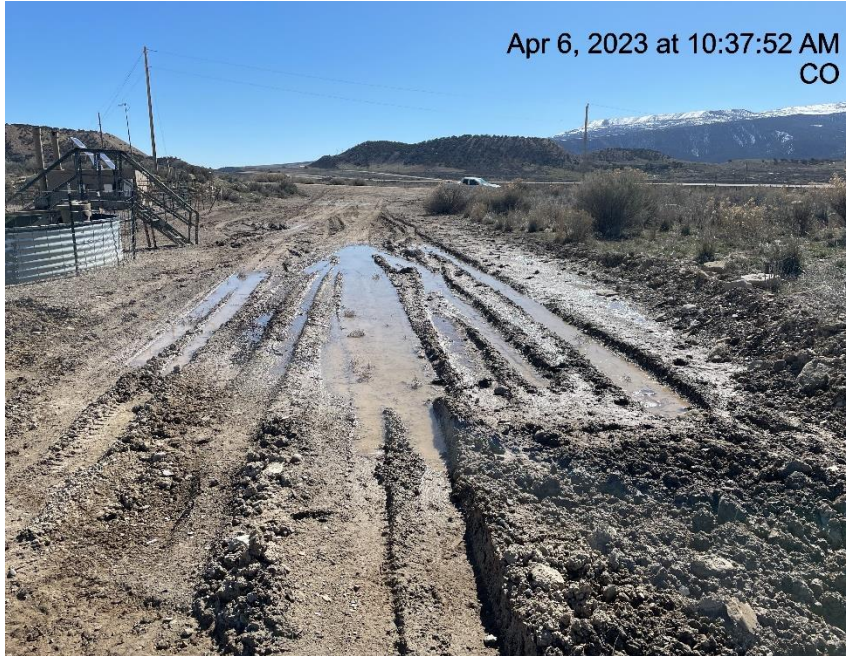
Photo # 4484 Lack of stabilization/insufficient tracking BMP's
