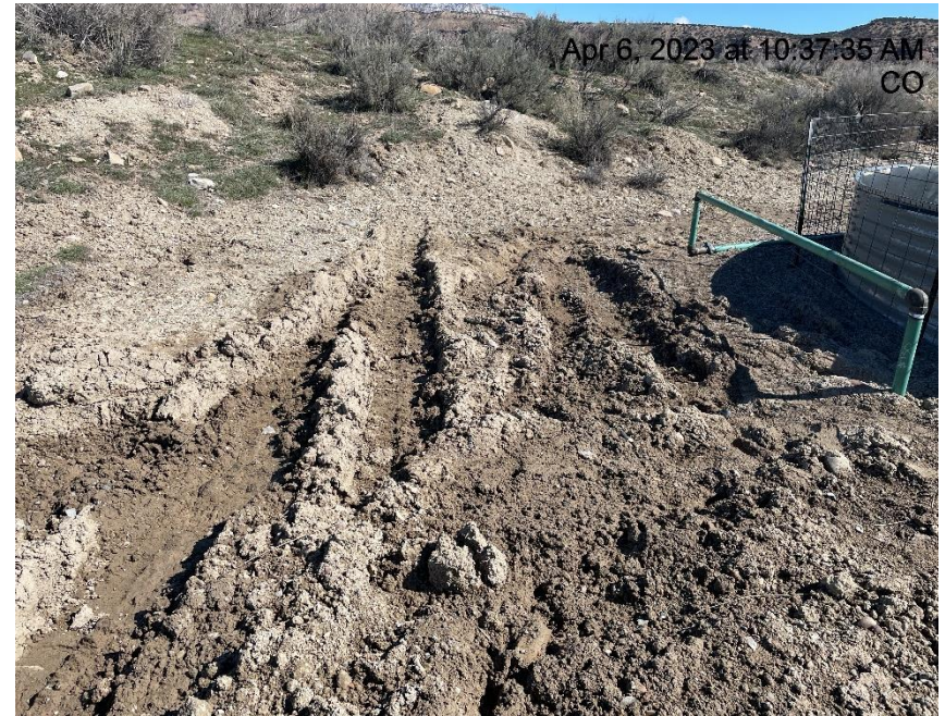
Photo # 4483 Lack of stabilization/compaction
