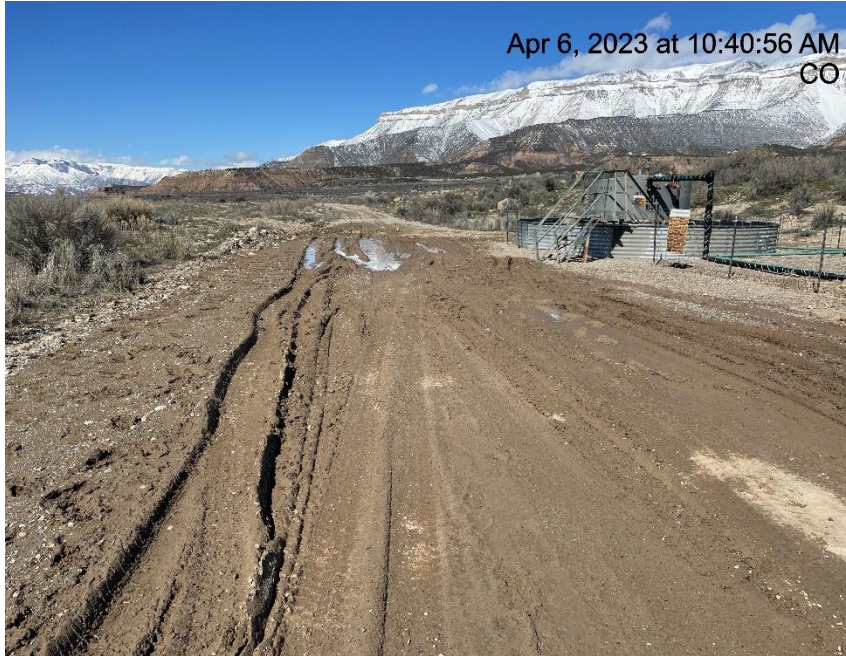
Photo # 4491 Lack of stabilization/insufficient tracking BMP's
