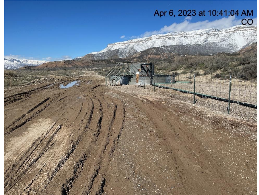
Photo # 4492 Lack of stabilization/insufficient tracking BMP's
