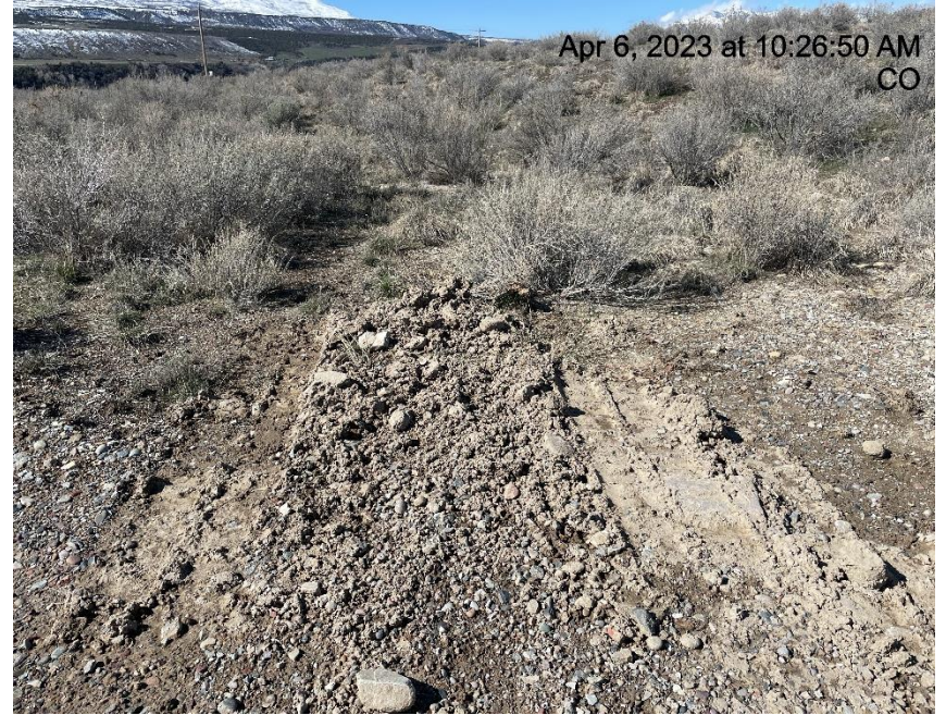
Photo # 4472 Failure to minimize surface disturbance/vehicle tracks into interim area/transport of sediment.
