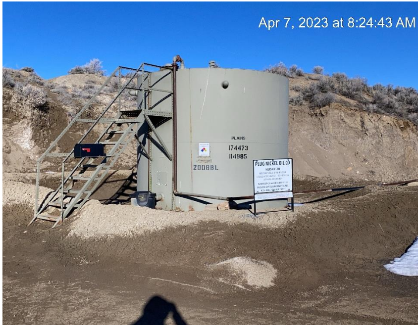
Tank battery with earth berm
