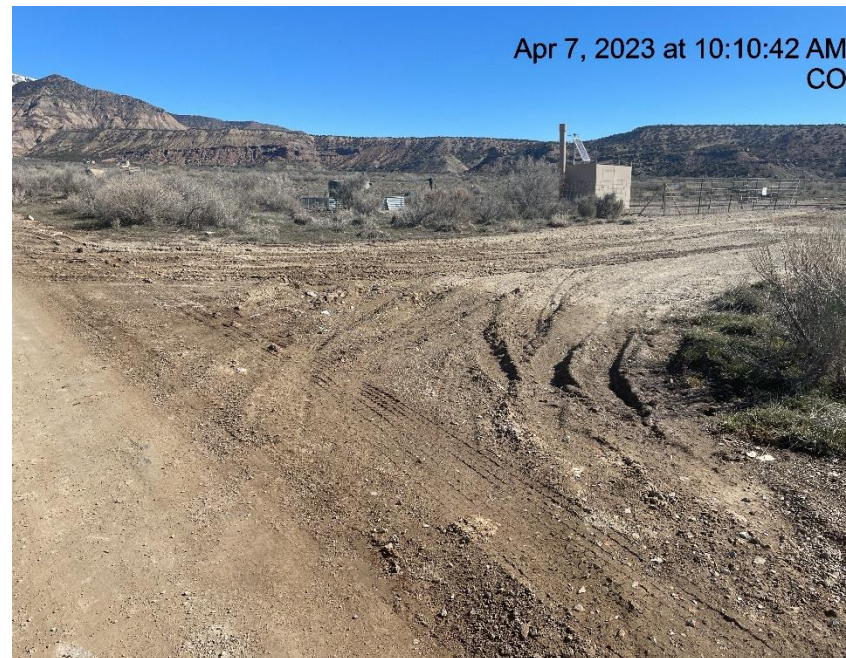
Photo # 4524 Lack of stabilization/Insufficient tracking BMP's/vehicle tracking
