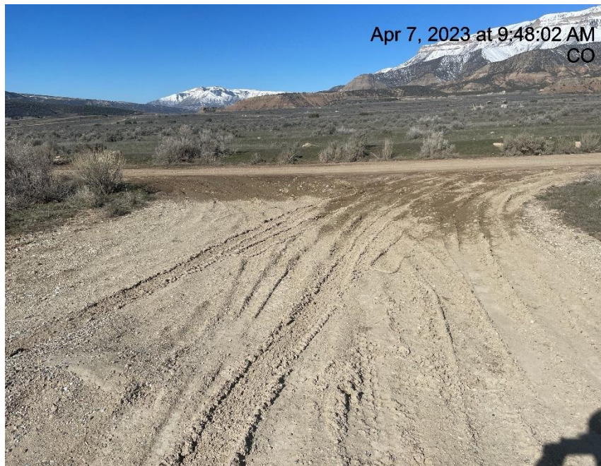
Photo # 4520 Lack of stabilization/Insufficient tracking BMP's
