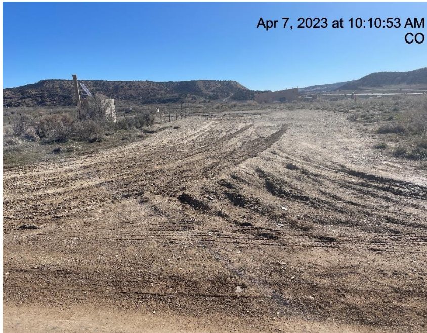
Photo # 4525 Lack of stabilization/Insufficient tracking BMP's
