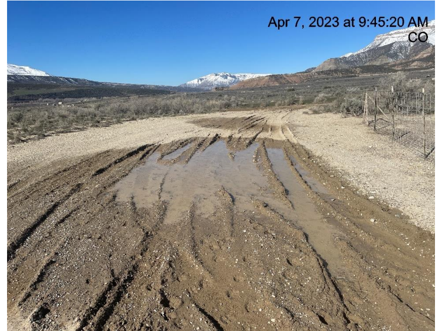
Photo # 4514 Lack of stabilization/Insufficient tracking BMP's
