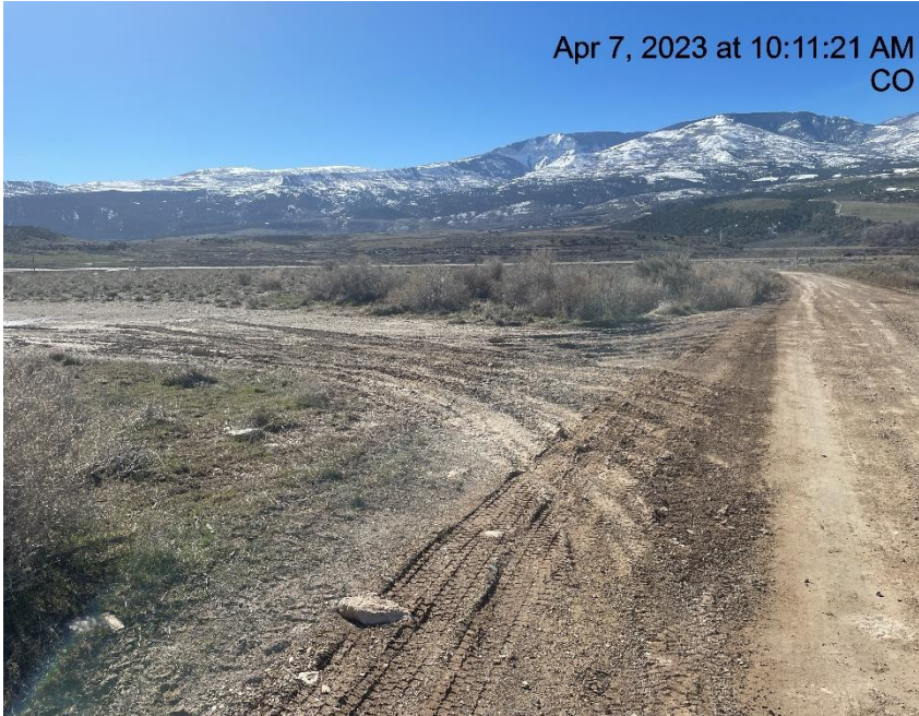
Photo # 4527 Vehicle tracking/Insufficient tracking BMP's
