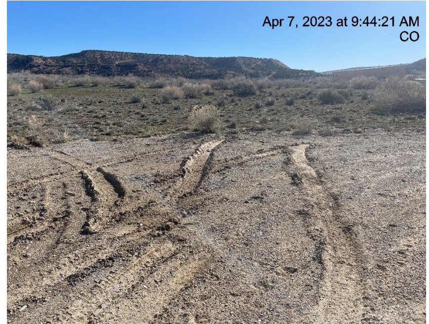
Photo # 4510 Lack of stabilization/Insufficient tracking BMP's
