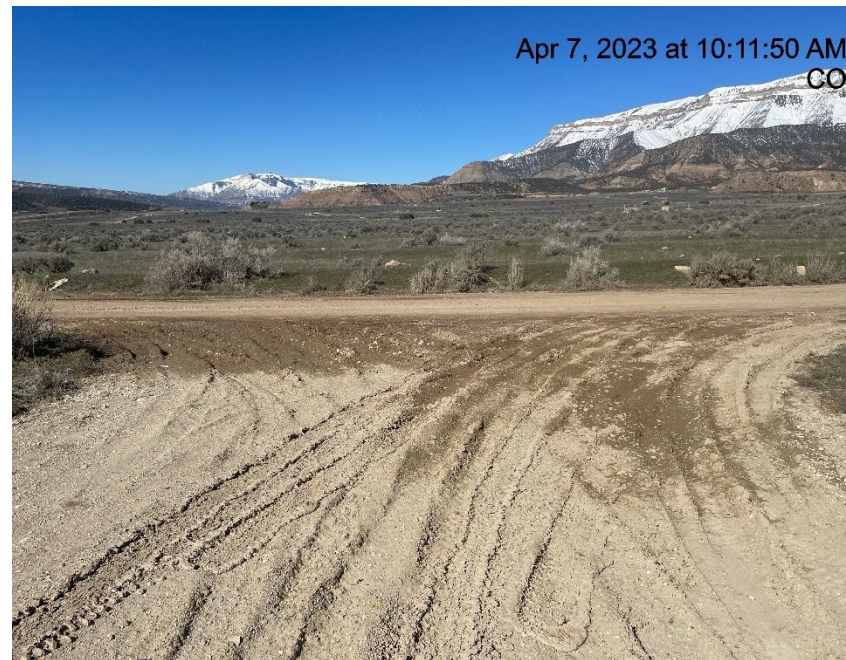
Photo # 4521 Lack of stabilization/Insufficient tracking BMP's
