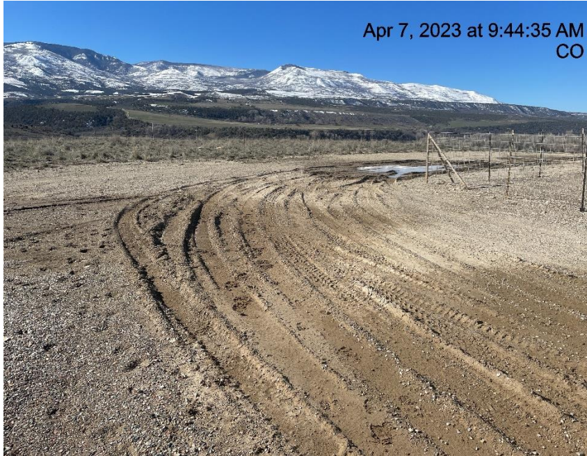
Photo # 4511 Lack of stabilization/Insufficient tracking BMP's
