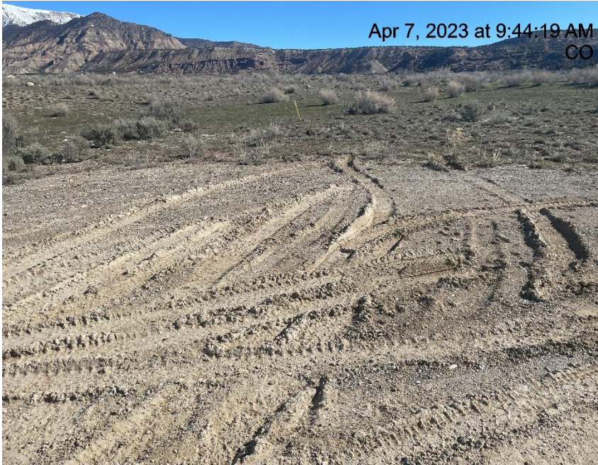
Photo # 4509 Lack of stabilization/Insufficient tracking BMP's
