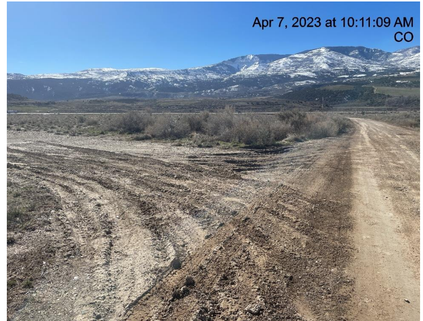
Photo # 4526 Vehicle tracking/Insufficient tracking BMP's
