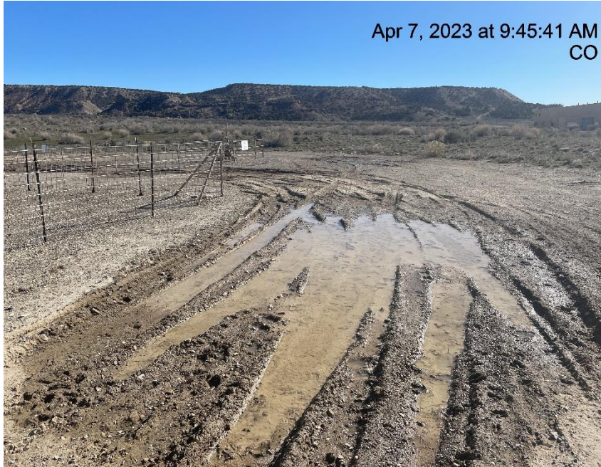
Photo # 4515 Lack of stabilization/Insufficient tracking BMP's
