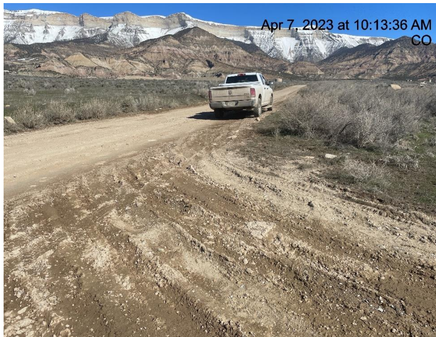
Photo # 4522 Lack of stabilization/Insufficient tracking BMP's
