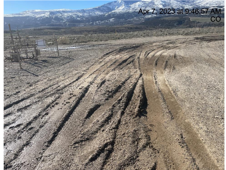
Photo # 4518 Lack of stabilization/Insufficient tracking BMP's
