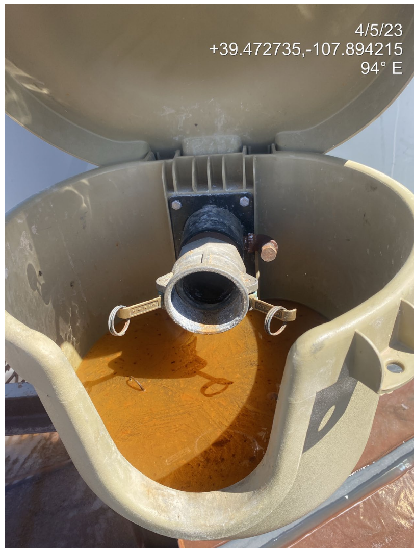
Photo 2. Photo shows a load line missing a bull plug/cap.
