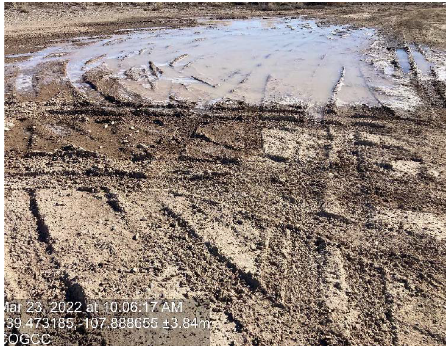
Photo 8. Photos show lack of stabilization/compaction from previous inspection (left) and current inspection (right).
