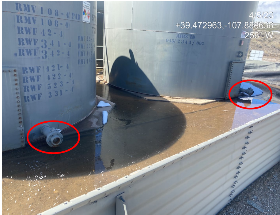
Photo 4. Photo shows bull plugs not installed on tank drain lines.
