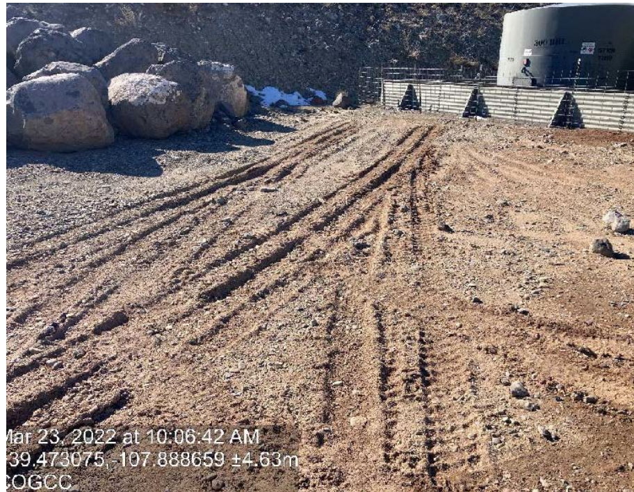
Photo 7. Photos show lack of stabilization/compaction from previous inspection (left) and current inspection (right).
