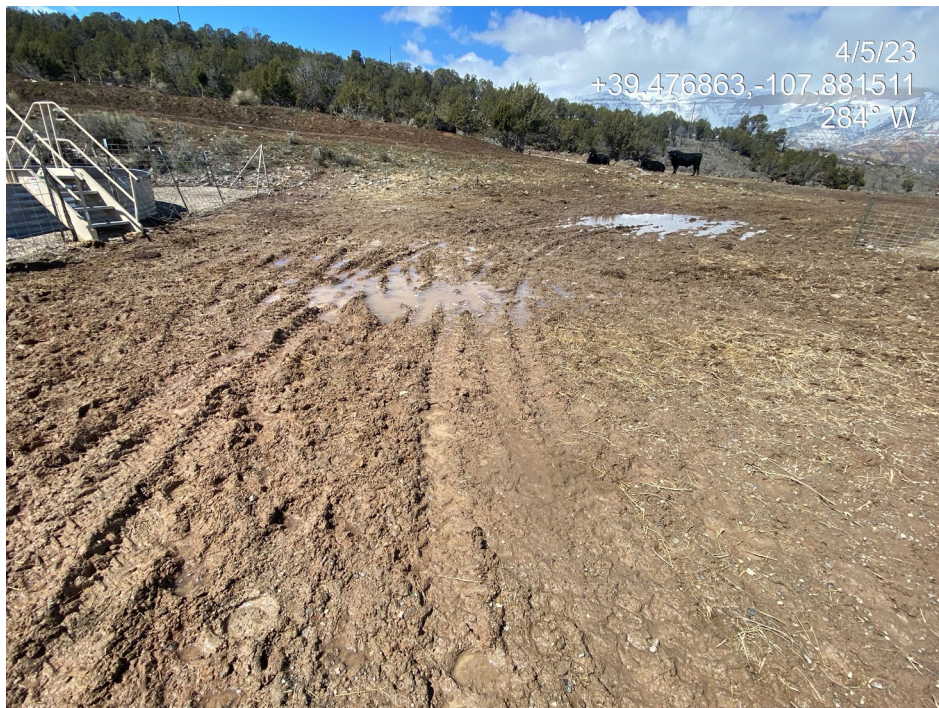
Photo 3. Photos show lack of stabilization of the pad surface.
