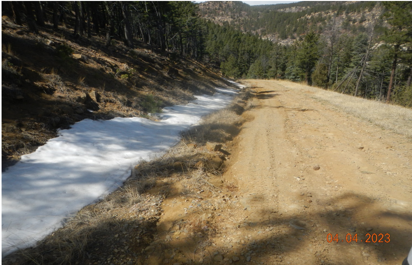
Photo 1. Facing northwest along the access road. There are culverts filled in with sediment along the portion of the road sand stormwater is causing erosion of the road.
