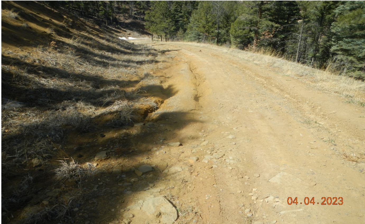
Photo 2. Facing northwest along the access road. There are culverts filled in with sediment along the portion of the road sand stormwater is causing erosion of the road.
